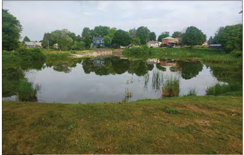
WILLS Saugeen Conservation Filename: 20230706_080546.jpg Photo 164 - October 26, 2023 Durham Creek Flood Plain Mapping Saugeen River: Lower Durham Dam Reservoir
