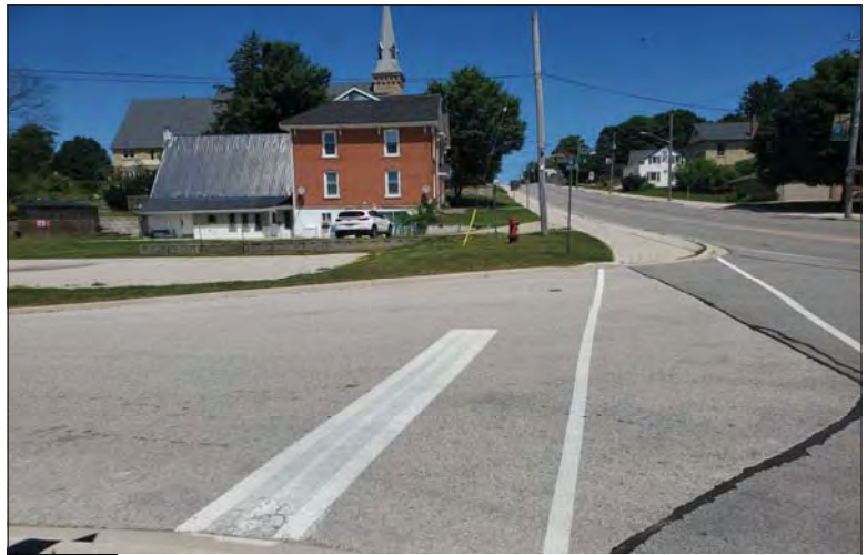
WILLS Saugeen Conservation Filename: 20230707_122601.jpg Photo 194 - October 26, 2023 Durham Creek Flood Plain Mapping Saugeen River: Highway 6 Bridge North Abutment Looking North
