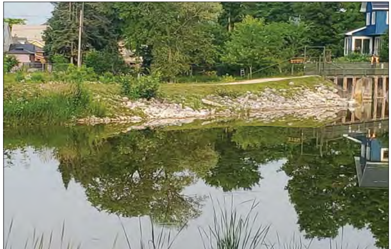
WILLS Saugeen Conservation Filename: 20230706_080627.jpg Photo 166 - October 26, 2023 Durham Creek Flood Plain Mapping Saugeen River: Lower Durham Dam Upstream Side of Earth Berm
