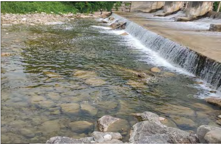
WILLS Saugeen Conservation Filename: 20230706_081120.jpg Photo 169 - October 26, 2023 Durham Creek Flood Plain Mapping Saugeen River: Lower Durham Dam Immediately Downstream
