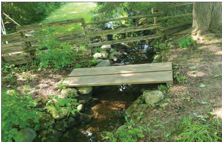
WILLS Saugeen Conservation Filename: 20230705_101052.jpg Photo 49 - October 26, 2023 Durham Creek Flood Plain Mapping Durham Creek: 245 Queen St S Backyard Footbridge Upstream Face
