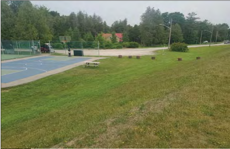
WILLS Saugeen Conservation Filename: 20230706_113309.jpg Photo 331 - October 26, 2023 Durham Creek Flood Plain Mapping Saugeen River: Upper Durham Dam South of Earth Berm
