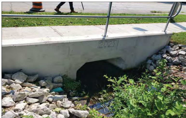
WILLS Saugeen Conservation Filename: 20230705_112548.jpg Photo 64 - October 26, 2023 Durham Creek Flood Plain Mapping Durham Creek: Garafraxa St S Culvert Downstream Face
