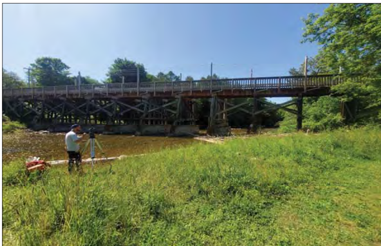
WILLS Saugeen Conservation Filename: 20230707_105916.jpg Photo 211 - October 26, 2023 Durham Creek Flood Plain Mapping Saugeen River: Heritage Walkway Bridge Upstream Face
