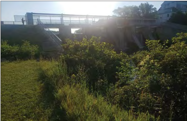
WILLS Saugeen Conservation Filename: 20230707_075341.jpg Photo 243 - October 26, 2023 Durham Creek Flood Plain Mapping Saugeen River: Middle Durham Dam Downstream Face
