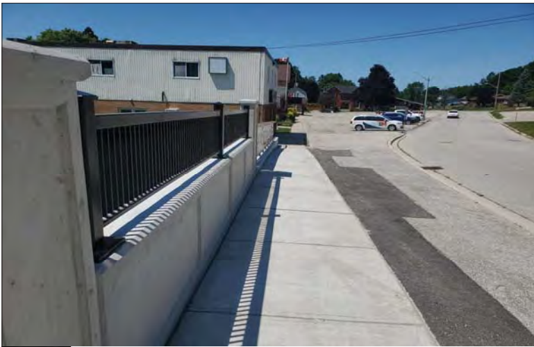
WILLS Saugeen Conservation Filename: 20230707_122557.jpg Photo 193 - October 26, 2023 Durham Creek Flood Plain Mapping Saugeen River: Highway 6 Bridge North Abutment Looking West Along George St W
