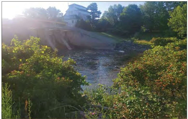
WILLS Saugeen Conservation Filename: 20230707_075349.jpg Photo 246 - October 26, 2023 Durham Creek Flood Plain Mapping Saugeen River: Middle Durham Dam Looking at Downstream South Bank
