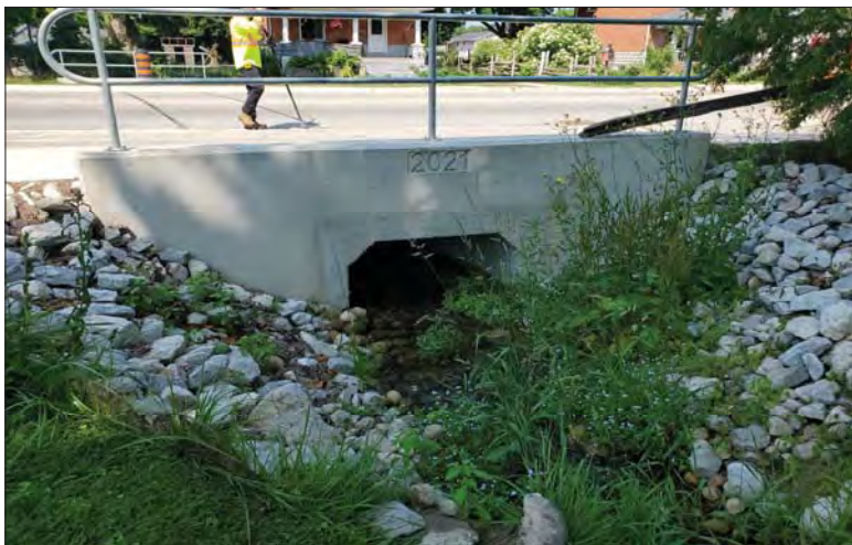
WILLS Saugeen Conservation Filename: 20230705_112443.jpg Photo 61 - October 26, 2023 Durham Creek Flood Plain Mapping Durham Creek: Garafraxa St S Culvert Upstream Face
