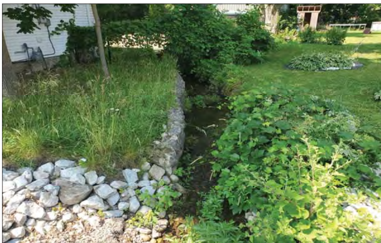
WILLS Saugeen Conservation Filename: 20230705_112558.jpg Photo 63 - October 26, 2023 Durham Creek Flood Plain Mapping Durham Creek: Garafraxa St S Culvert Looking Downstream
