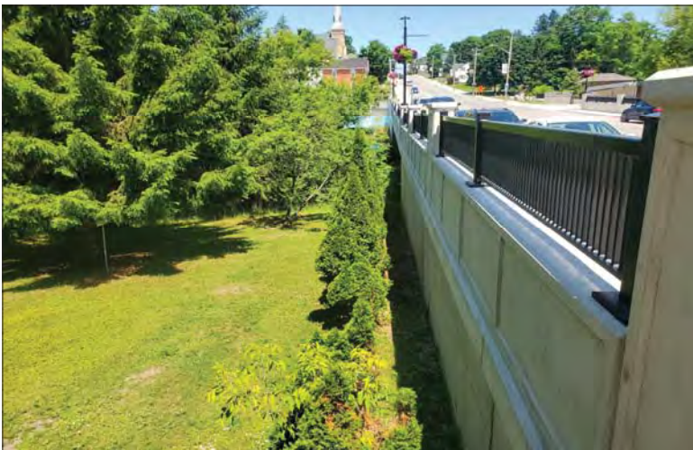
WILLS Saugeen Conservation Filename: 20230707_122929.jpg Photo 191 - October 26, 2023 Durham Creek Flood Plain Mapping Saugeen River: Highway 6 Bridge Downstream Face
