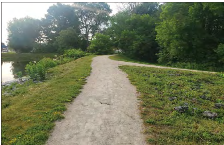
WILLS Saugeen Conservation Filename: 20230706_080227.jpg Photo 141 - October 26, 2023 Durham Creek Flood Plain Mapping Saugeen River: Lower Durham Dam Earth Berm
