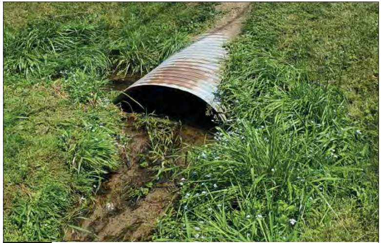
WILLS Saugeen Conservation Filename: 20230704_131455.jpg Photo 16 - October 26, 2023 Durham Creek Flood Plain Mapping Durham Creek: Queen St S Downstream Face
