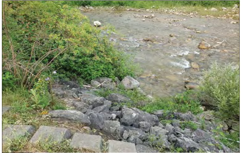
WILLS Saugeen Conservation Filename: 20230706_081029.jpg Photo 152 - October 26, 2023 Durham Creek Flood Plain Mapping Saugeen River: Lower Durham Dam End of Emergency Spillway
