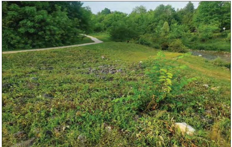
WILLS Saugeen Conservation Filename: 20230706_080249.jpg Photo 148 - October 26, 2023 Durham Creek Flood Plain Mapping Saugeen River: Lower Durham Dam Emergency Spillway
