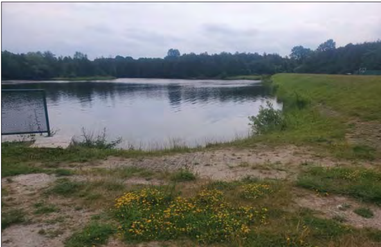
WILLS Saugeen Conservation Filename: 20230706_111536.jpg Photo 285 - October 26, 2023 Durham Creek Flood Plain Mapping Saugeen River: Upper Durham Dam Looking Upstream
