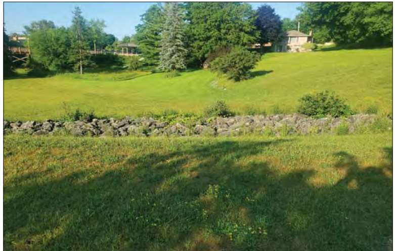
WILLS Saugeen Conservation Filename: 20230707_080215.jpg Photo 238 - October 26, 2023 Durham Creek Flood Plain Mapping Saugeen River: Middle Durham Dam Looking Southwest
