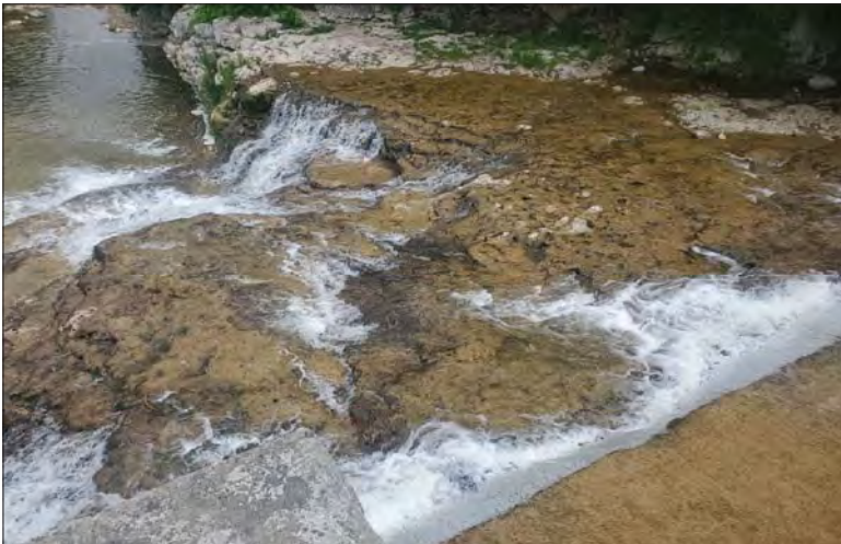
WILLS Saugeen Conservation Filename: 20230706_111825.jpg Photo 303 - October 26, 2023 Durham Creek Flood Plain Mapping Saugeen River: Upper Durham Dam Immediately Downstream
