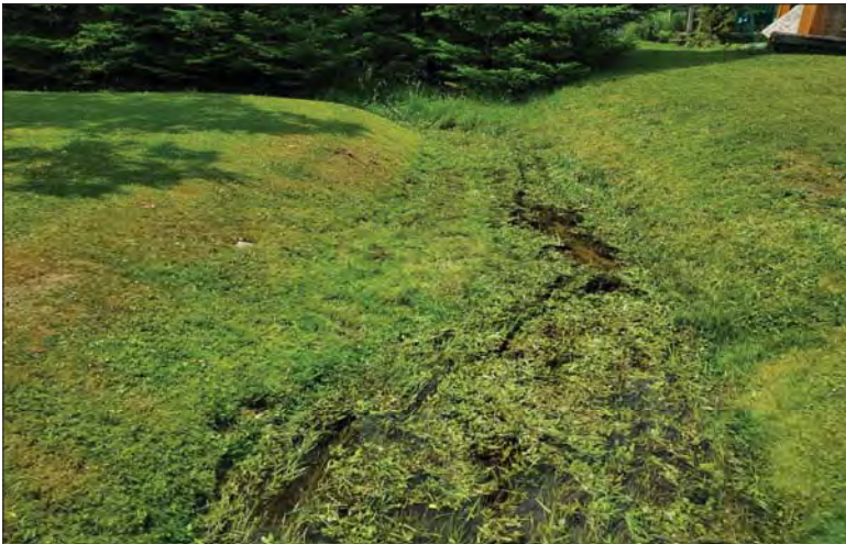
WILLS Saugeen Conservation Filename: 20230705_131054.jpg Photo 75 - October 26, 2023 Durham Creek Flood Plain Mapping Durham Creek: 197 Saddler St E Backyard Footbridge Looking Downstream
