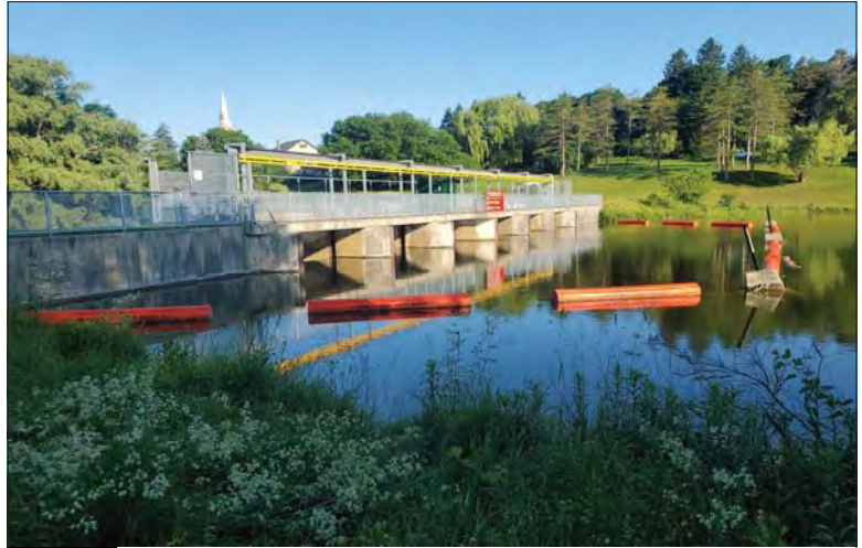
WILLS Saugeen Conservation Filename: 20230707_081324.jpg Photo 236 - October 26, 2023 Durham Creek Flood Plain Mapping Saugeen River: Middle Durham Dam Upstream Face
