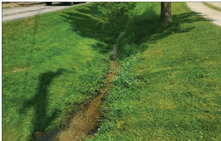
WILLS Saugeen Conservation Filename: 20230705_145634.jpg Photo 98 - October 26, 2023 Durham Creek Flood Plain Mapping Durham Creek: Elgin St S Culvert Looking Upstream
