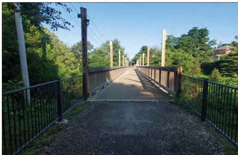
WILLS Saugeen Conservation Filename: 20230707_081519.jpg Photo 214 - October 26, 2023 Durham Creek Flood Plain Mapping Saugeen River: Heritage Walkway Bridge East Abutment Looking West
