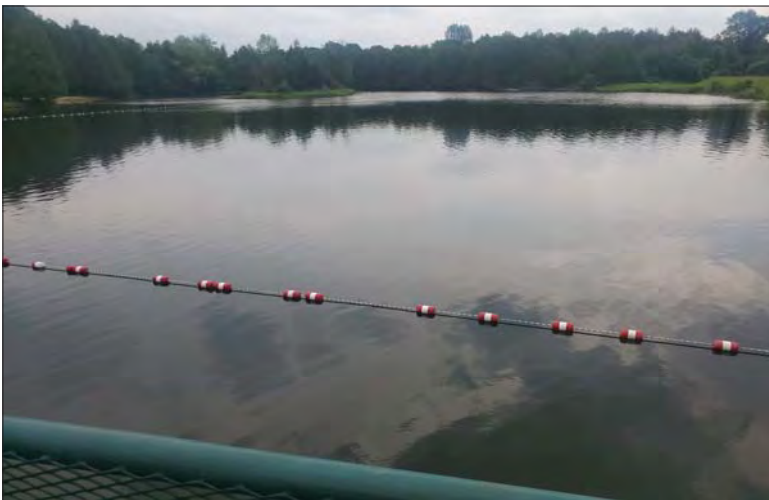
WILLS Saugeen Conservation Filename: 20230706_111656.jpg Photo 293 - October 26, 2023 Durham Creek Flood Plain Mapping Saugeen River: Upper Durham Dam Looking Upstream
