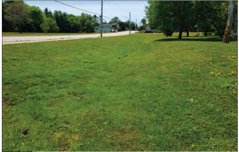
WILLS Saugeen Conservation Filename: 20230707_143837.jpg Photo 116 - October 26, 2023 Durham Creek Flood Plain Mapping Durham Creek: Grey County Rd 4 Culvert Upstream Looking West
