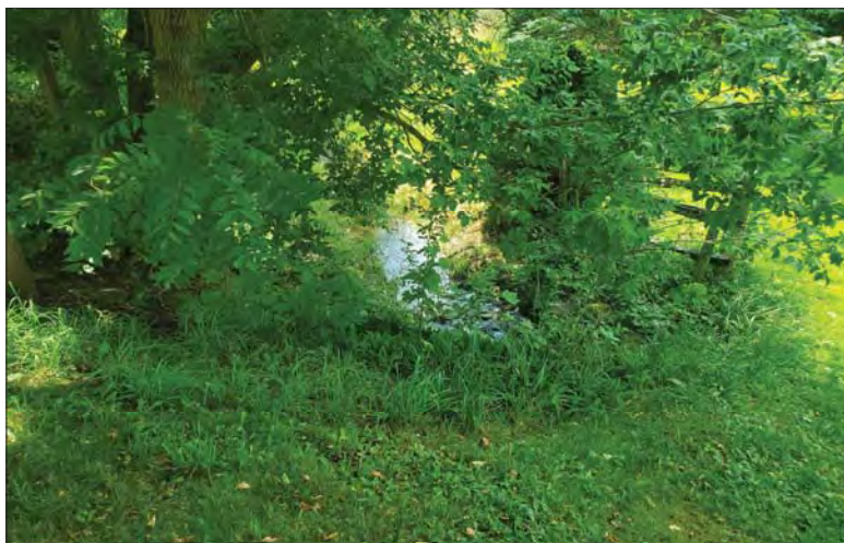
WILLS Saugeen Conservation Filename: 20230705_153204.jpg Photo 105 - October 26, 2023 Durham Creek Flood Plain Mapping Durham Creek: Kincardine St S Culvert Looking Downstream
