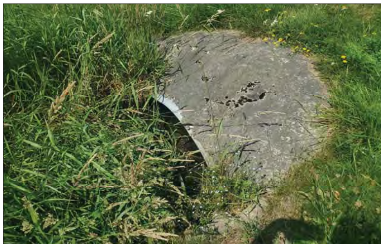
WILLS Saugeen Conservation Filename: 20230705_145718.jpg Photo 100 - October 26, 2023 Durham Creek Flood Plain Mapping Durham Creek: Elgin St S Culvert Downstream Face
