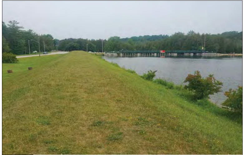
WILLS Saugeen Conservation Filename: 20230706_113312.jpg Photo 332 - October 26, 2023 Durham Creek Flood Plain Mapping Saugeen River: Upper Durham Dam Earth Berm
