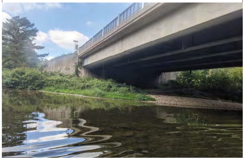
WILLS Saugeen Conservation Filename: PXL_20230914_161825667.jpg Photo 2 - September 14, 2023 Durham Creek Flood Plain Mapping Saugeen River: Grey County Road 4 Bridge Upstream Soffit and West Wingwall
