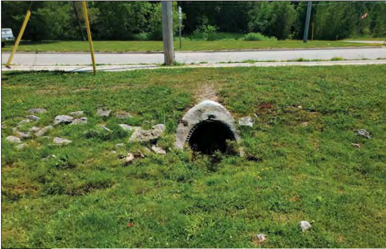
WILLS Saugeen Conservation Filename: 20230707_143833.jpg Photo 115 - October 26, 2023 Durham Creek Flood Plain Mapping Durham Creek: Grey County Rd 4 Culvert Upstream Face
