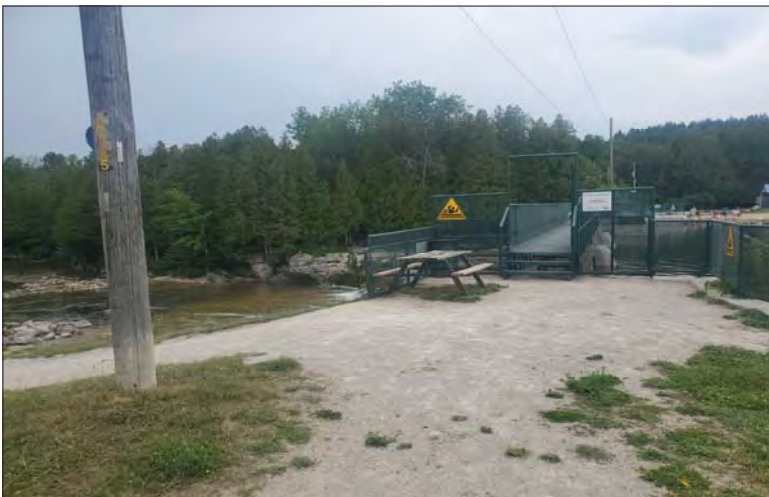
WILLS Saugeen Conservation Filename: 20230706_111604.jpg Photo 287 - October 26, 2023 Durham Creek Flood Plain Mapping Saugeen River: Upper Durham Dam
