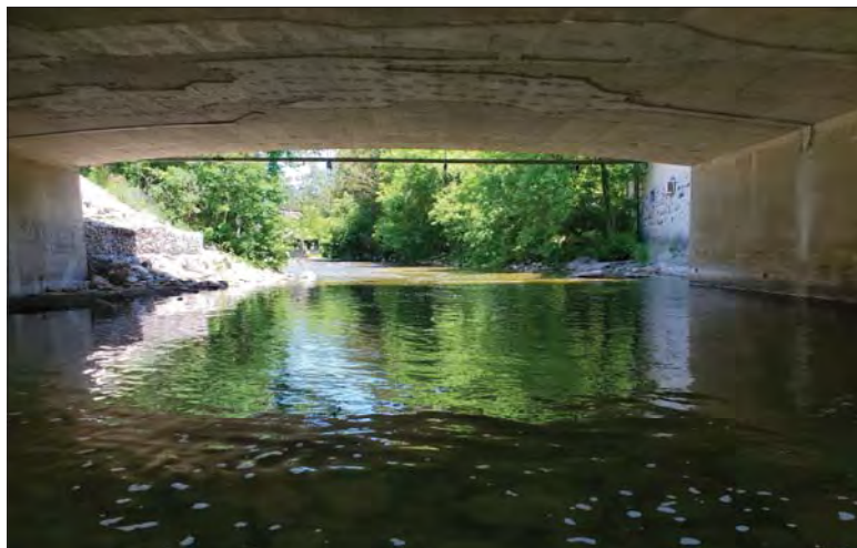
WILLS Saugeen Conservation Filename: 20230707_134142.jpg Photo 206 - October 26, 2023 Durham Creek Flood Plain Mapping Saugeen River: Highway 6 Bridge Soffit Looking Upstream
