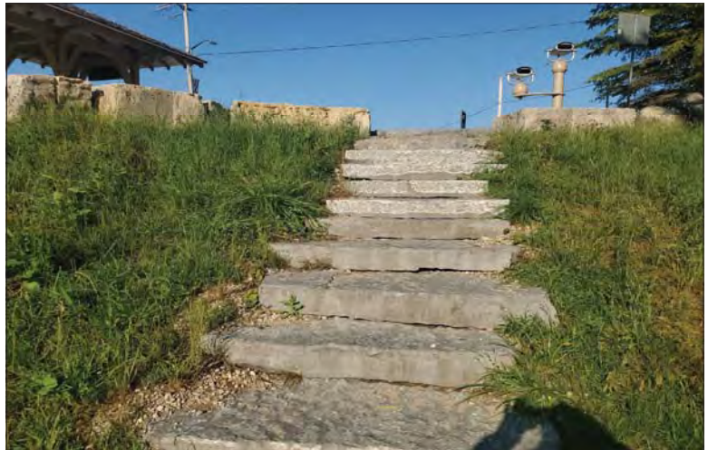
WILLS Saugeen Conservation Filename: 20230707_081825.jpg Photo 226 - October 26, 2023 Durham Creek Flood Plain Mapping Saugeen River: Heritage Walkway Bridge West Stairs to River
