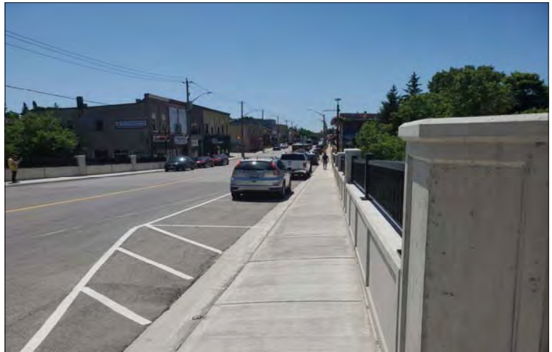
WILLS Saugeen Conservation Filename: 20230707_122612.jpg Photo 196 - October 26, 2023 Durham Creek Flood Plain Mapping Saugeen River: Highway 6 Bridge North Abutment Looking South
