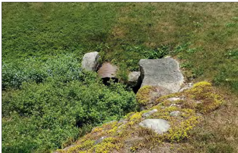
WILLS Saugeen Conservation Filename: 20230705_131937.jpg Photo 85 - October 26, 2023 Durham Creek Flood Plain Mapping Durham Creek: Saddler St E Culvert Upstream Face
