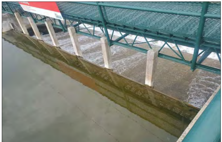
WILLS Saugeen Conservation Filename: 20230706_111805.jpg Photo 300 - October 26, 2023 Durham Creek Flood Plain Mapping Saugeen River: Upper Durham Dam Upstream Face of Middle Spillway
