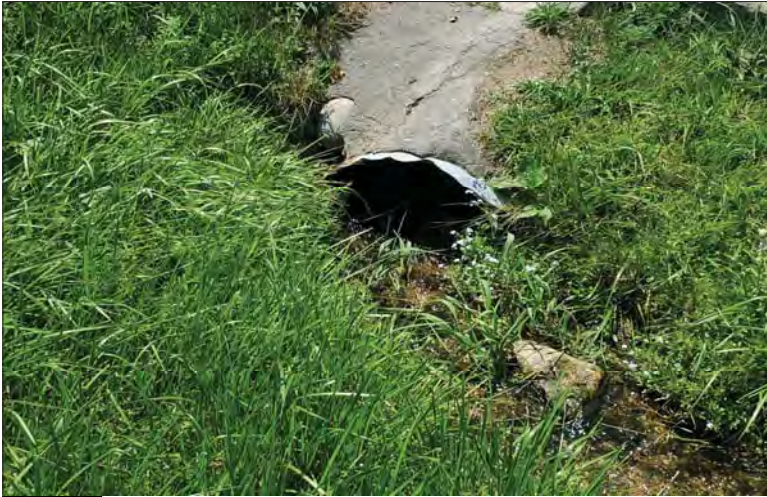
WILLS Saugeen Conservation Filename: 20230704_131413.jpg Photo 13 - October 26, 2023 Durham Creek Flood Plain Mapping Durham Creek: Queen St S Upstream Face
