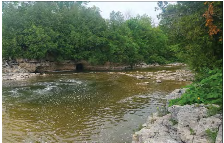
WILLS Saugeen Conservation Filename: 20230706_112930.jpg Photo 320 - October 26, 2023 Durham Creek Flood Plain Mapping Saugeen River: Upper Durham Dam Downstream South Bank
