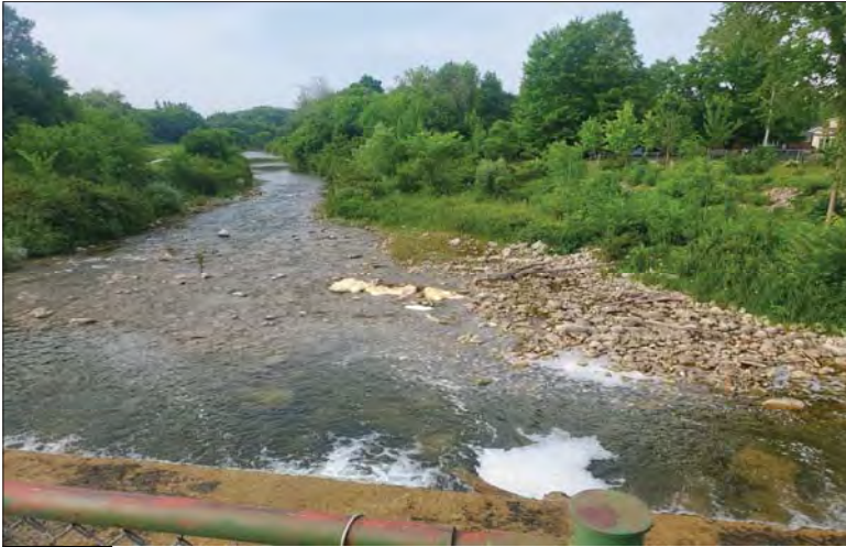
WILLS Saugeen Conservation Filename: 20230706_080117.jpg Photo 133 - October 26, 2023 Durham Creek Flood Plain Mapping Saugeen River: Lower Durham Dam Looking Downstream
