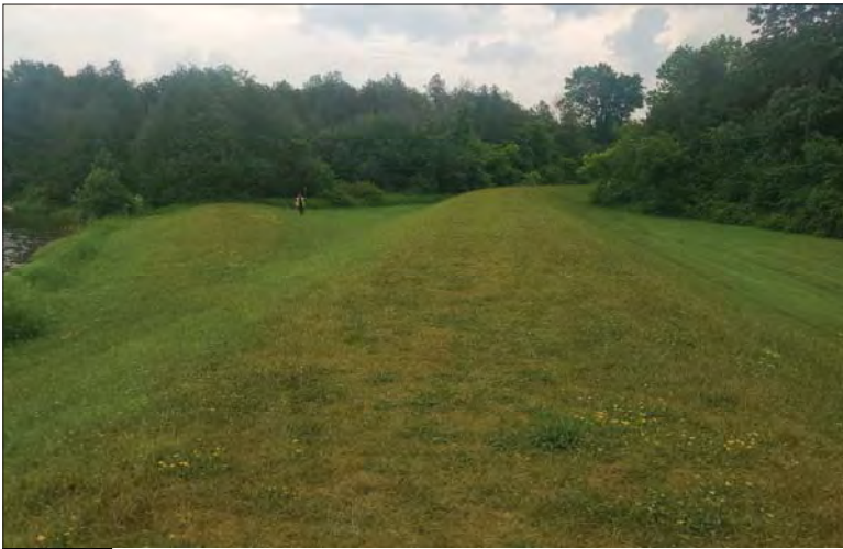
WILLS Saugeen Conservation Filename: 20230706_113303.jpg Photo 329 - October 26, 2023 Durham Creek Flood Plain Mapping Saugeen River: Upper Durham Dam Earth Berm
