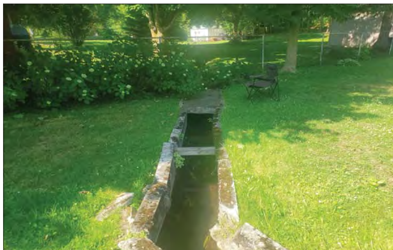
WILLS Saugeen Conservation Filename: 20230704_163750.jpg Photo 34 - October 26, 2023 Durham Creek Flood Plain Mapping Durham Creek: 265 Queen St S Backyard Channel Looking Upstream
