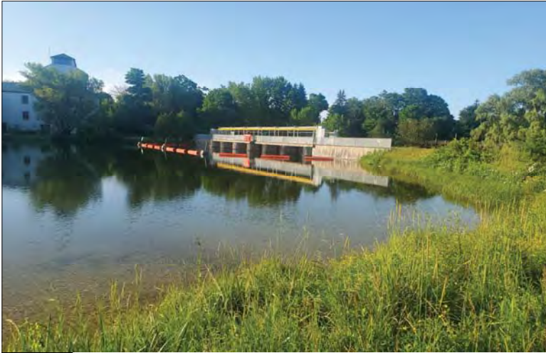
WILLS Saugeen Conservation Filename: 20230707_080256.jpg Photo 235 - October 26, 2023 Durham Creek Flood Plain Mapping Saugeen River: Middle Durham Dam Upstream Face
