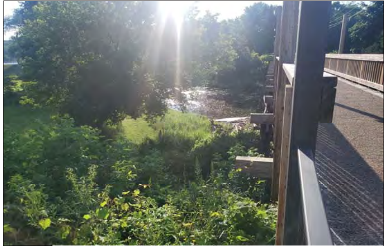
WILLS Saugeen Conservation Filename: 20230707_081748.jpg Photo 224 - October 26, 2023 Durham Creek Flood Plain Mapping Saugeen River: Heritage Walkway Bridge
