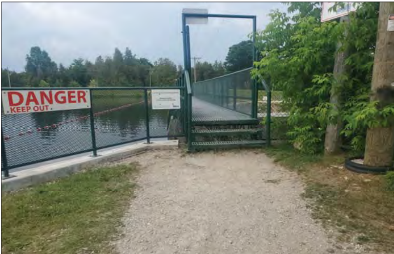
WILLS Saugeen Conservation Filename: 20230706_111925.jpg Photo 309 - October 26, 2023 Durham Creek Flood Plain Mapping Saugeen River: Upper Durham Dam North End of Deck
