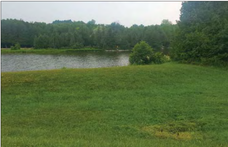
WILLS Saugeen Conservation Filename: 20230706_113503.jpg Photo 339 - October 26, 2023 Durham Creek Flood Plain Mapping Saugeen River: Upper Durham Dam Earth Berm Looking North at Overflow Pipe
