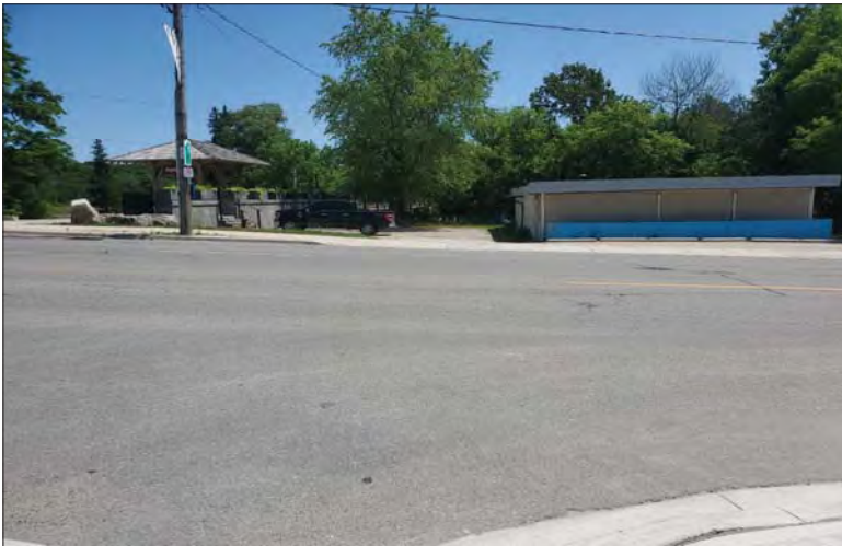
WILLS Saugeen Conservation Filename: 20230707_122604.jpg Photo 195 - October 26, 2023 Durham Creek Flood Plain Mapping Saugeen River: Highway 6 Bridge North Abutment Looking East
