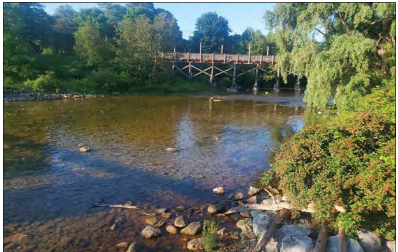
WILLS Saugeen Conservation Filename: 20230707_075503.jpg Photo 248 - October 26, 2023 Durham Creek Flood Plain Mapping Saugeen River: Middle Durham Dam Looking Downstream
