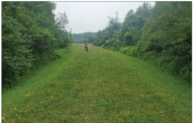
WILLS Saugeen Conservation Filename: 20230706_113930.jpg Photo 342 - October 26, 2023 Durham Creek Flood Plain Mapping Saugeen River: Upper Durham Dam Earth Berm South of Reservoir Looking North
