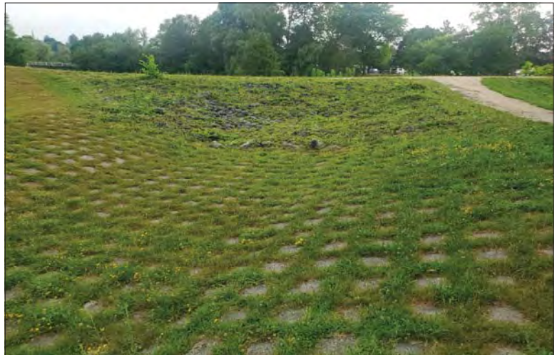
WILLS Saugeen Conservation Filename: 20230706_080902.jpg Photo 150 - October 26, 2023 Durham Creek Flood Plain Mapping Saugeen River: Lower Durham Dam Emergency Spillway
