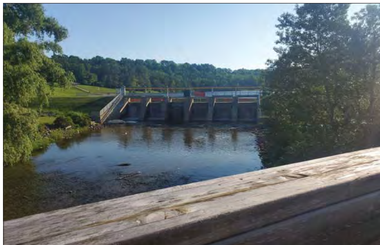
WILLS Saugeen Conservation Filename: 20230707_081601.jpg Photo 212 - October 26, 2023 Durham Creek Flood Plain Mapping Saugeen River: Heritage Walkway Bridge Looking Upstream
