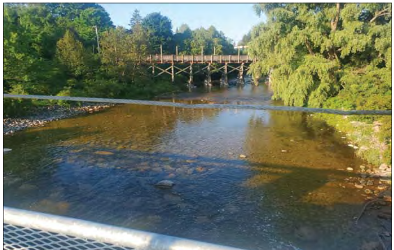
WILLS Saugeen Conservation Filename: 20230707_075654.jpg Photo 252 - October 26, 2023 Durham Creek Flood Plain Mapping Saugeen River: Middle Durham Dam Looking Downstream
