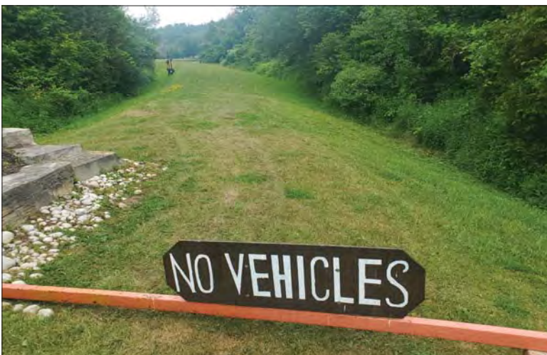
WILLS Saugeen Conservation Filename: 20230706_114006.jpg Photo 347 - October 26, 2023 Durham Creek Flood Plain Mapping Saugeen River: Upper Durham Dam Earth Berm South of Reservoir at End of Berm at Grey County Road 4
