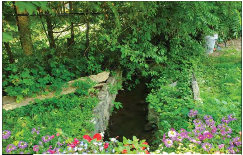
WILLS Saugeen Conservation Filename: 20230705_123026.jpg Photo 70 - October 26, 2023 Durham Creek Flood Plain Mapping Durham Creek: 232 Garafraxa St S Driveway Culvert Looking Downstream
