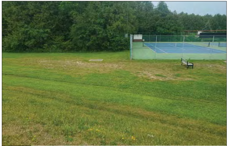
WILLS Saugeen Conservation Filename: 20230706_113306.jpg Photo 330 - October 26, 2023 Durham Creek Flood Plain Mapping Saugeen River: Upper Durham Dam South of Earth Berm
