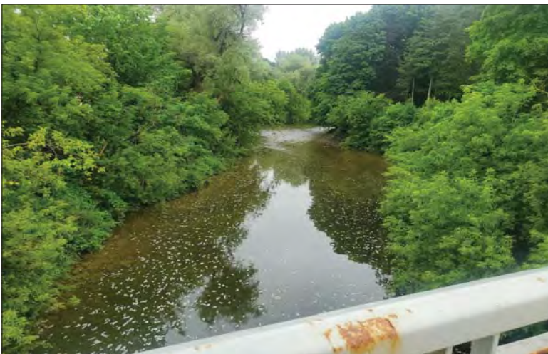
WILLS Saugeen Conservation Filename: 20230706_154325.jpg Photo 179 - October 26, 2023 Durham Creek Flood Plain Mapping Saugeen River: Lambton St E Bridge Looking Upstream
