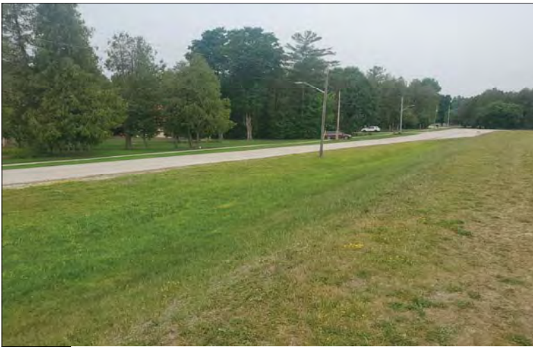
WILLS Saugeen Conservation Filename: 20230706_113209.jpg Photo 325 - October 26, 2023 Durham Creek Flood Plain Mapping Saugeen River: Upper Durham Dam South of Earth Berm
