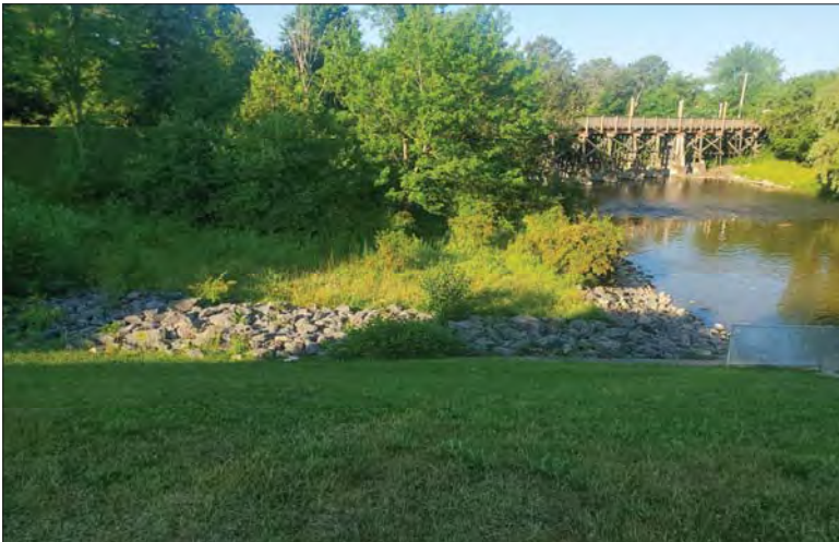
WILLS Saugeen Conservation Filename: 20230707_075908.jpg Photo 267 - October 26, 2023 Durham Creek Flood Plain Mapping Saugeen River: Middle Durham Dam Looking Downstream from South Bank
