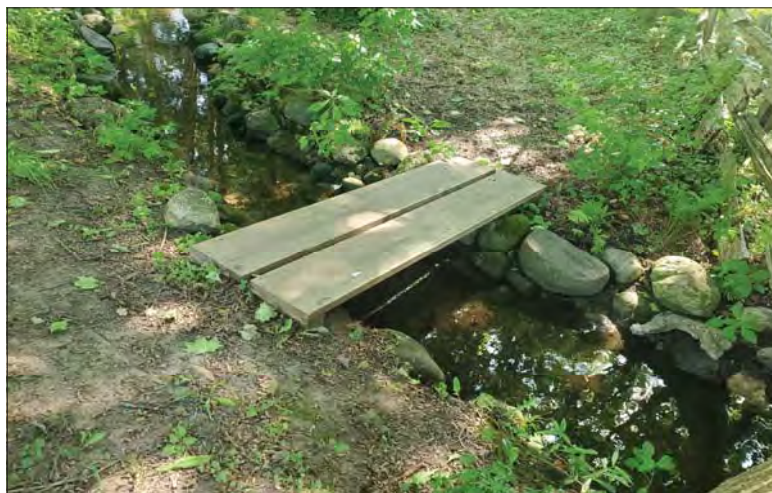
WILLS Saugeen Conservation Filename: 20230705_101114.jpg Photo 52 - October 26, 2023 Durham Creek Flood Plain Mapping Durham Creek: 245 Queen St S Backyard Footbridge Downstream Face
