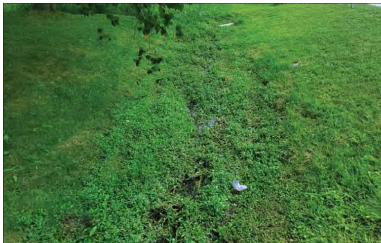
WILLS Saugeen Conservation Filename: 20230705_133939.jpg Photo 92 - October 26, 2023 Durham Creek Flood Plain Mapping Durham Creek: 242 Saddler St E Driveway Culvert Looking Upstream
