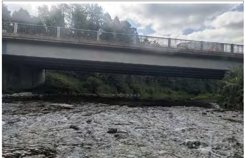
WILLS Saugeen Conservation Filename: PXL_20230914_161732619.jpg Photo 6 - September 14, 2023 Durham Creek Flood Plain Mapping Saugeen River: Grey County Road 4 Bridge Downstream Face
