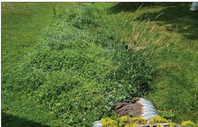
WILLS Saugeen Conservation Filename: 20230705_133951.jpg Photo 93 - October 26, 2023 Durham Creek Flood Plain Mapping Durham Creek: 242 Saddler St E Driveway Culvert Looking Downstream
