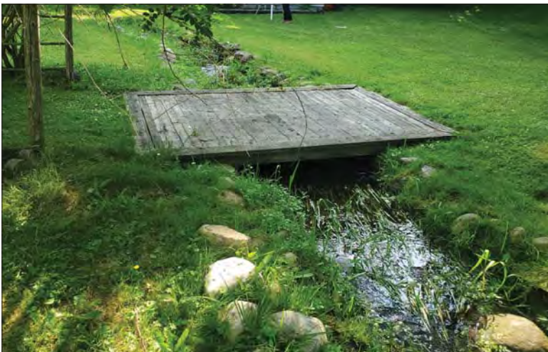
WILLS Saugeen Conservation Filename: 20230705_092802.jpg Photo 41 - October 26, 2023 Durham Creek Flood Plain Mapping Durham Creek: 249 Queen St S Backyard Footbridge 1 Downstream Face
