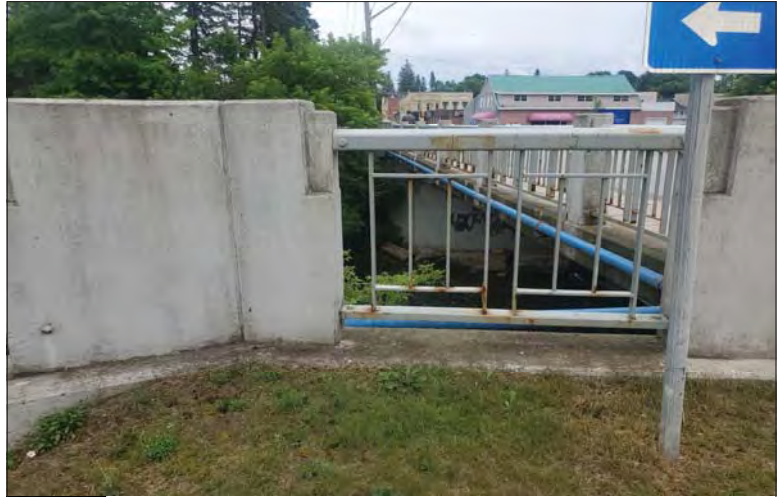
WILLS Saugeen Conservation Filename: 20230706_154405.jpg Photo 176 - October 26, 2023 Durham Creek Flood Plain Mapping Saugeen River: Lambton St E Bridge Upstream Face and West Wingwall
