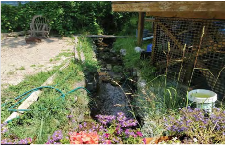
WILLS Saugeen Conservation Filename: 20230705_123017.jpg Photo 69 - October 26, 2023 Durham Creek Flood Plain Mapping Durham Creek: 232 Garafraxa St S Driveway Culvert Looking Upstream
