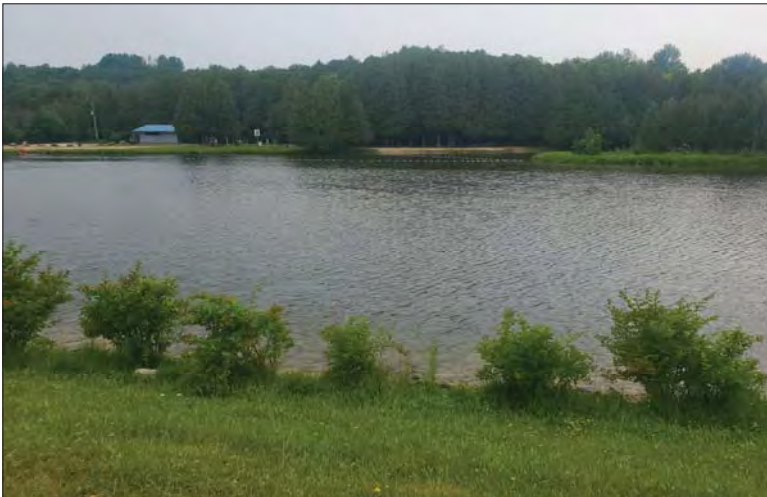
WILLS Saugeen Conservation Filename: 20230706_113315.jpg Photo 333 - October 26, 2023 Durham Creek Flood Plain Mapping Saugeen River: Upper Durham Dam View from Earth Berm
