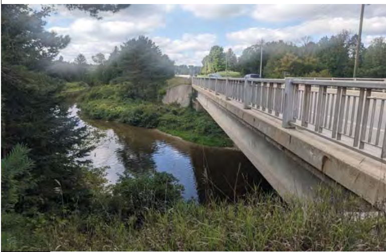
WILLS Saugeen Conservation Filename: PXL_20230914_161914005.jpg Photo 1 - September 14, 2023 Durham Creek Flood Plain Mapping Saugeen River: Grey County Road 4 Bridge Upstream Face
