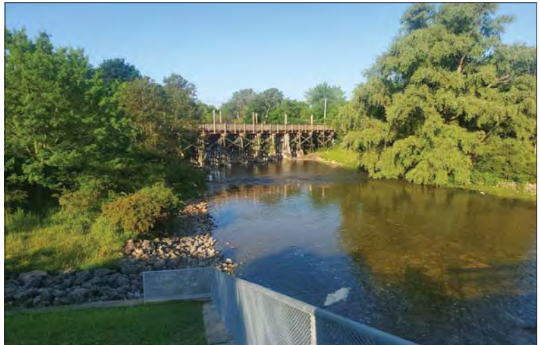
WILLS Saugeen Conservation Filename: 20230707_080018.jpg Photo 268 - October 26, 2023 Durham Creek Flood Plain Mapping Saugeen River: Middle Durham Dam Looking Downstream
