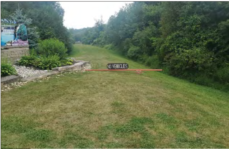
Filename: 20230706_114205.jpg Photo 349 - October 26, 2023 Durham Creek Flood Plain Mapping Saugeen River: Upper Durham Dam Earth Berm South of Reservoir at End of Berm at Grey County Road 4
