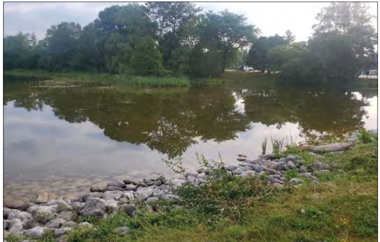
WILLS Saugeen Conservation Filename: 20230706_080232.jpg Photo 142 - October 26, 2023 Durham Creek Flood Plain Mapping Saugeen River: Lower Durham Dam Reservoir
