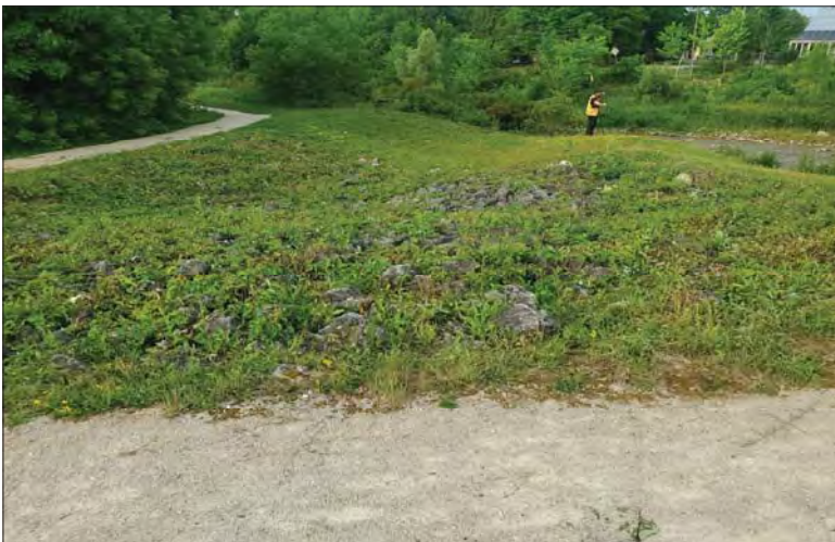
WILLS Saugeen Conservation Filename: 20230706_080803.jpg Photo 147 - October 26, 2023 Durham Creek Flood Plain Mapping Saugeen River: Lower Durham Dam Emergency Spillway
