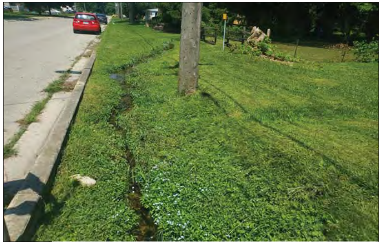
WILLS Saugeen Conservation Filename: 20230704_133425.jpg Photo 20 - October 26, 2023 Durham Creek Flood Plain Mapping Durham Creek: 295 Queen St S Driveway Looking Upstream
