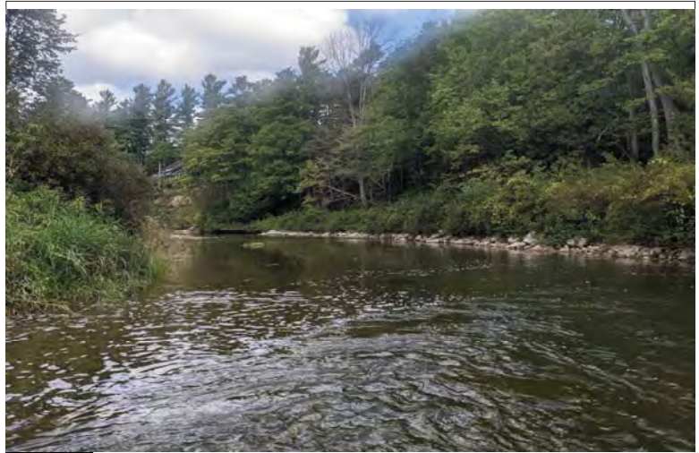
WILLS Saugeen Conservation Filename: PXL_20230914_161738066.jpg Photo 8 - September 14, 2023 Durham Creek Flood Plain Mapping Saugeen River: Grey County Road 4 Bridge Looking Downstream
