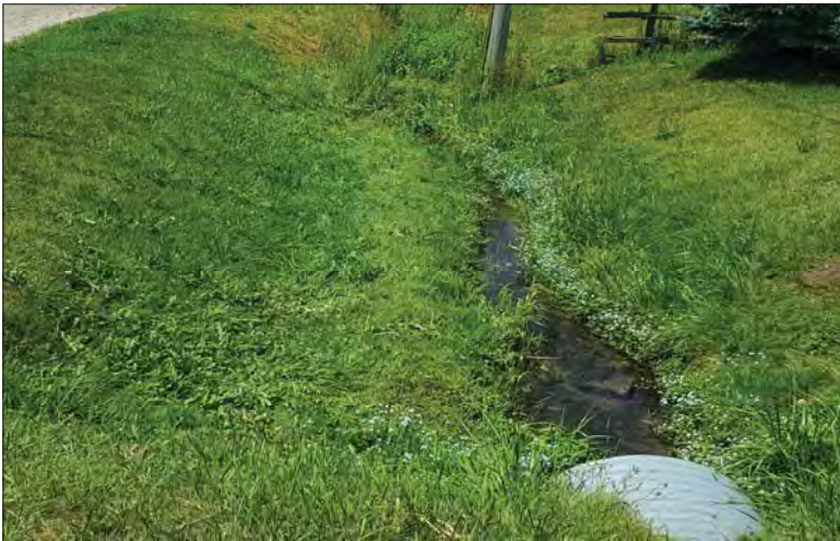
WILLS Saugeen Conservation Filename: 20230704_125815.jpg Photo 9 - October 26, 2023 Durham Creek Flood Plain Mapping Durham Creek: 274 South St W Driveway Facing Downstream
