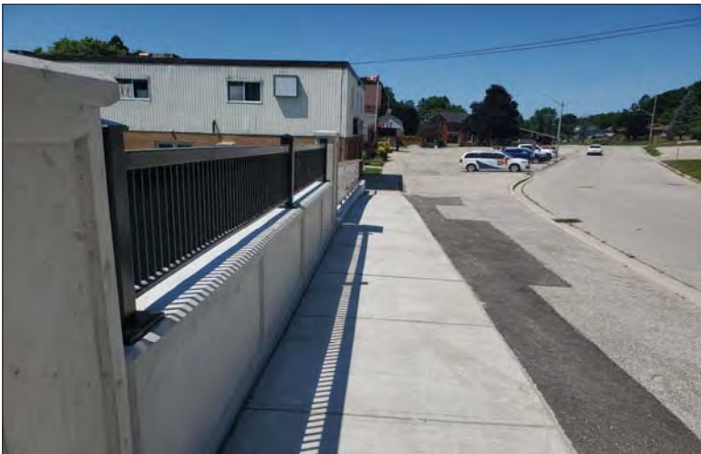
WILLS Saugeen Conservation Filename: 20230707_122557.jpg Photo 193 - October 26, 2023 Durham Creek Flood Plain Mapping Saugeen River: Highway 6 Bridge North Abutment Looking West Along George St W
