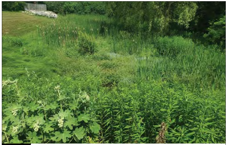
WILLS Saugeen Conservation Filename: 20230705_153051.jpg Photo 104 - October 26, 2023 Durham Creek Flood Plain Mapping Durham Creek: Kincardine St S Culvert Looking Upstream
