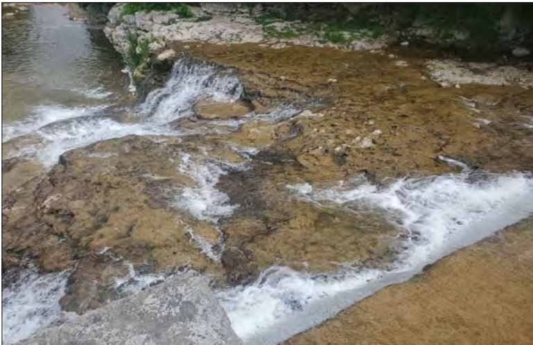
WILLS Saugeen Conservation Filename: 20230706_111825.jpg Photo 303 - October 26, 2023 Durham Creek Flood Plain Mapping Saugeen River: Upper Durham Dam Immediately Downstream
