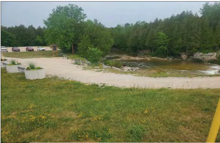
WILLS Saugeen Conservation Filename: 20230706_111524.jpg Photo 283 - October 26, 2023 Durham Creek Flood Plain Mapping Saugeen River: Upper Durham Dam Looking Downstream
