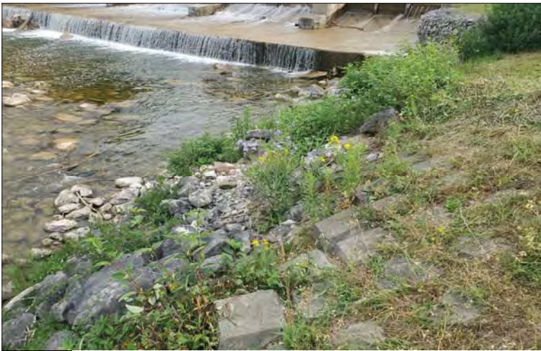
WILLS Saugeen Conservation Filename: 20230706_081019.jpg Photo 151 - October 26, 2023 Durham Creek Flood Plain Mapping Saugeen River: Lower Durham Dam End of Emergency Spillway
