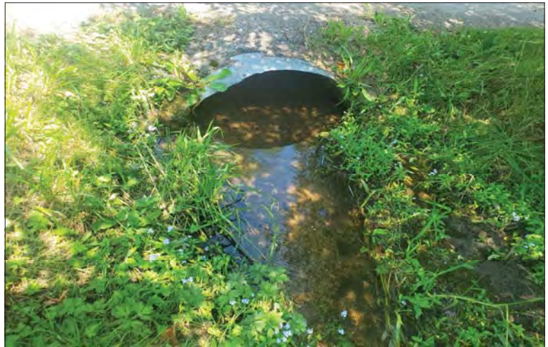
WILLS Saugeen Conservation Filename: 20230704_133445.jpg Photo 22 - October 26, 2023 Durham Creek Flood Plain Mapping Durham Creek: 295 Queen St S Driveway Downstream Face
