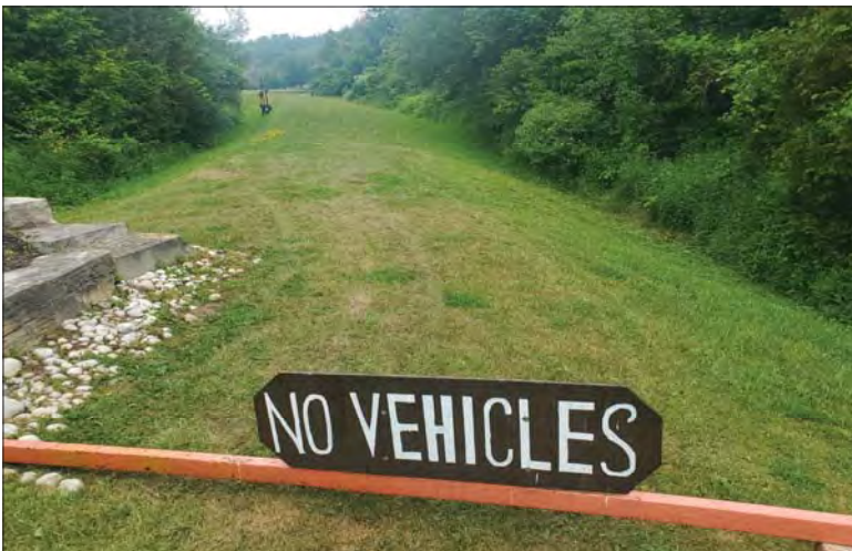
WILLS Saugeen Conservation Filename: 20230706_114006.jpg Photo 347 - October 26, 2023 Durham Creek Flood Plain Mapping Saugeen River: Upper Durham Dam Earth Berm South of Reservoir at End of Berm at Grey County Road 4
