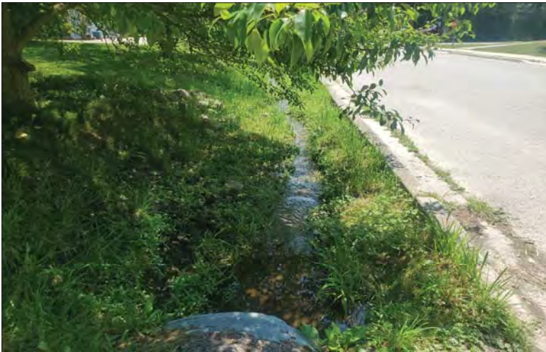
WILLS Saugeen Conservation Filename: 20230704_133433.jpg Photo 21 - October 26, 2023 Durham Creek Flood Plain Mapping Durham Creek: 295 Queen St S Driveway Looking Downstream
