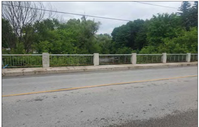
WILLS Saugeen Conservation Filename: 20230706_154214.jpg Photo 182 - October 26, 2023 Durham Creek Flood Plain Mapping Saugeen River: Lambton St E Bridge Looking North
