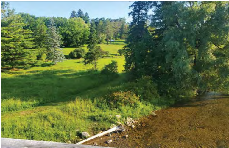
WILLS Saugeen Conservation Filename: 20230707_081650.jpg Photo 223 - October 26, 2023 Durham Creek Flood Plain Mapping Saugeen River: Heritage Walkway Bridge Looking North
