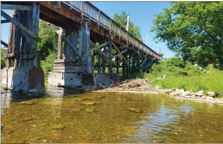
WILLS Saugeen Conservation Filename: 20230707_112808.jpg Photo 229 - October 26, 2023 Durham Creek Flood Plain Mapping Saugeen River: Heritage Walkway Bridge West Bank
