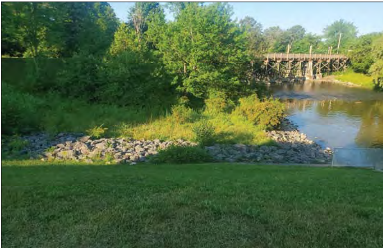
WILLS Saugeen Conservation Filename: 20230707_075908.jpg Photo 267 - October 26, 2023 Durham Creek Flood Plain Mapping Saugeen River: Middle Durham Dam Looking Downstream from South Bank
