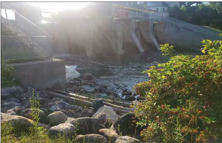
WILLS Saugeen Conservation Filename: 20230707_075420.jpg Photo 245 - October 26, 2023 Durham Creek Flood Plain Mapping Saugeen River: Middle Durham Dam Downstream Face
