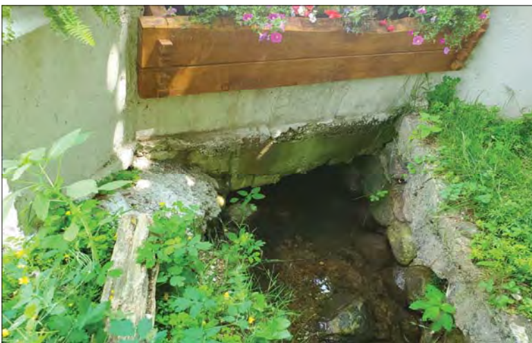
WILLS Saugeen Conservation Filename: 20230705_123037.jpg Photo 71 - October 26, 2023 Durham Creek Flood Plain Mapping Durham Creek: 232 Garafraxa St S Driveway Culvert Downstream Face
