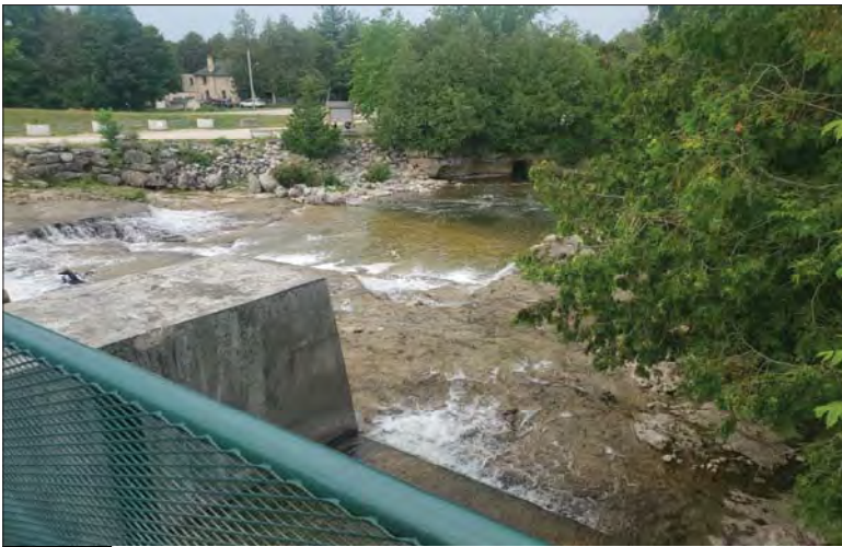
WILLS Saugeen Conservation Filename: 20230706_111910.jpg Photo 307 - October 26, 2023 Durham Creek Flood Plain Mapping Saugeen River: Upper Durham Dam Looking Downstream
