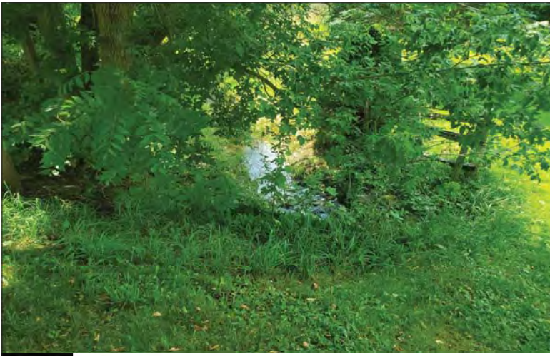
WILLS Saugeen Conservation Filename: 20230705_153204.jpg Photo 105 - October 26, 2023 Durham Creek Flood Plain Mapping Durham Creek: Kincardine St S Culvert Looking Downstream
