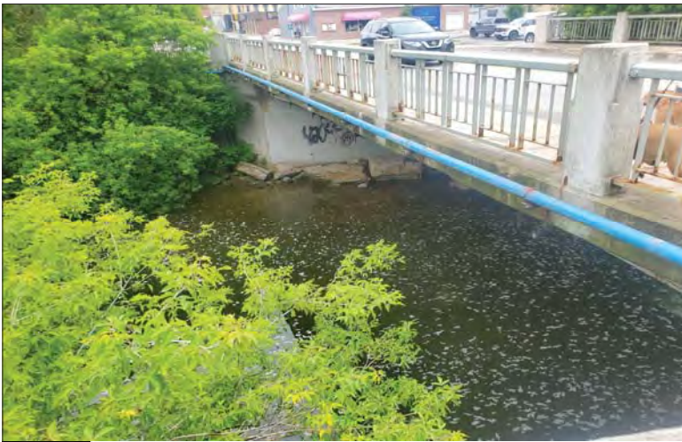
WILLS Saugeen Conservation Filename: 20230706_154354.jpg Photo 175 - October 26, 2023 Durham Creek Flood Plain Mapping Saugeen River: Lambton St E Bridge Upstream Face
