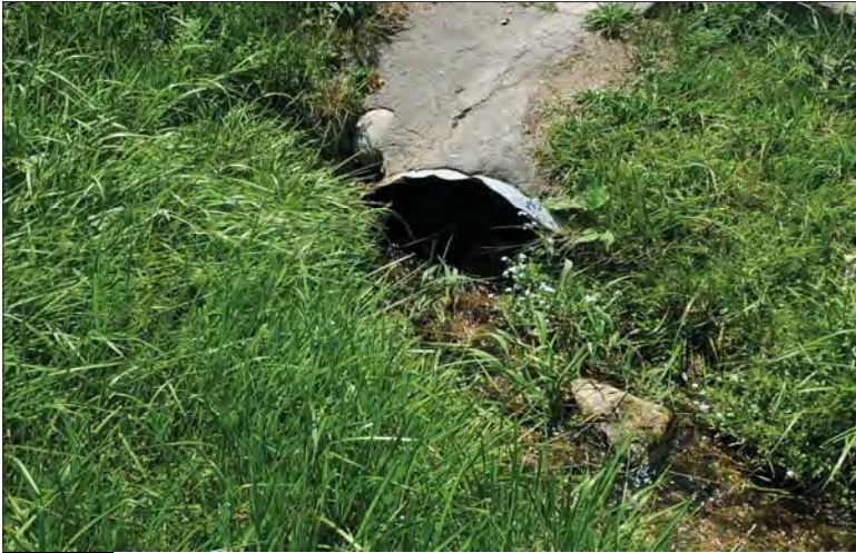
WILLS Saugeen Conservation Filename: 20230704_131413.jpg Photo 13 - October 26, 2023 Durham Creek Flood Plain Mapping Durham Creek: Queen St S Upstream Face
