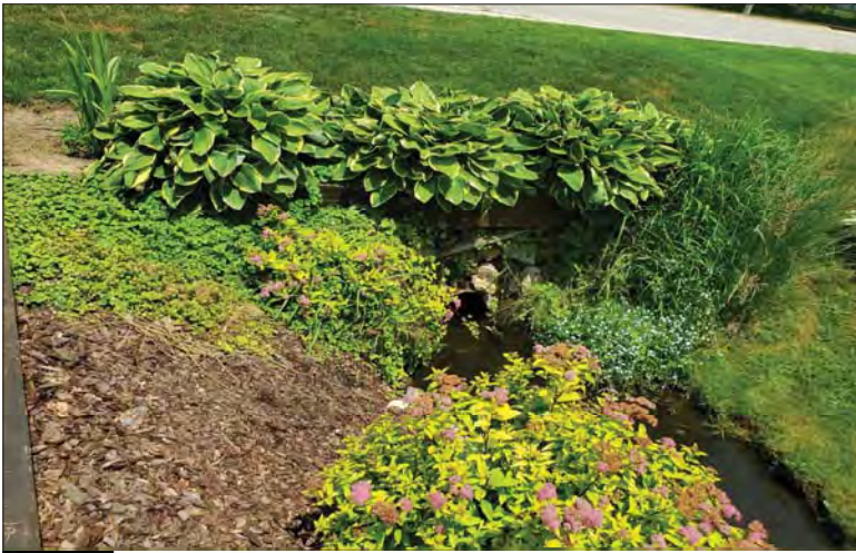
WILLS Saugeen Conservation Filename: 20230705_132031.jpg Photo 87 - October 26, 2023 Durham Creek Flood Plain Mapping Durham Creek: Saddler St E Culvert Downstream Face
