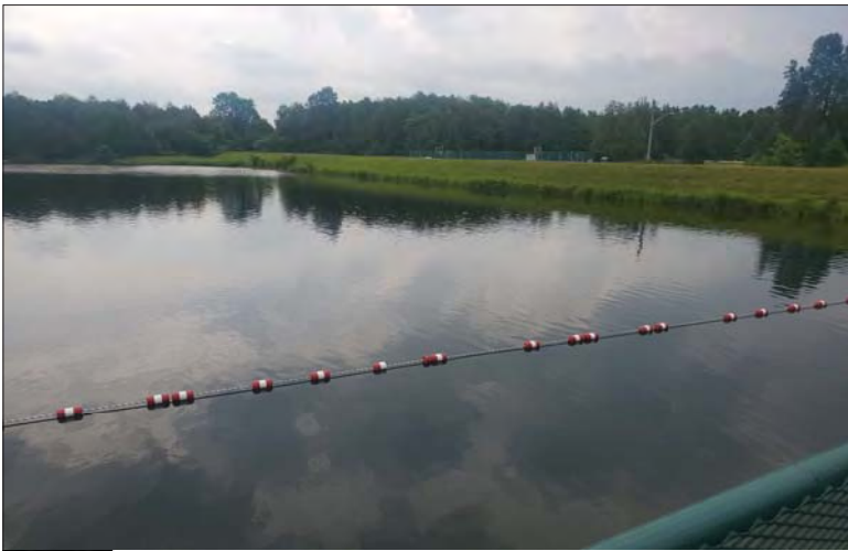
WILLS Saugeen Conservation Filename: 20230706_111719.jpg Photo 295 - October 26, 2023 Durham Creek Flood Plain Mapping Saugeen River: Upper Durham Dam Upstream South Bank and Earth Berm
