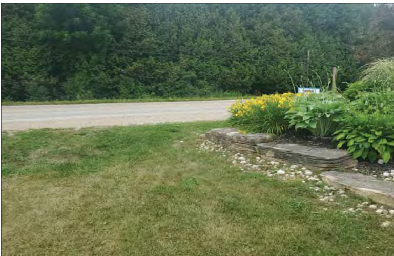
WILLS Saugeen Conservation Filename: 20230706_113956.jpg Photo 345 - October 26, 2023 Durham Creek Flood Plain Mapping Saugeen River: Upper Durham Dam Earth Berm South of Reservoir at End of Berm at Grey County Road 4
