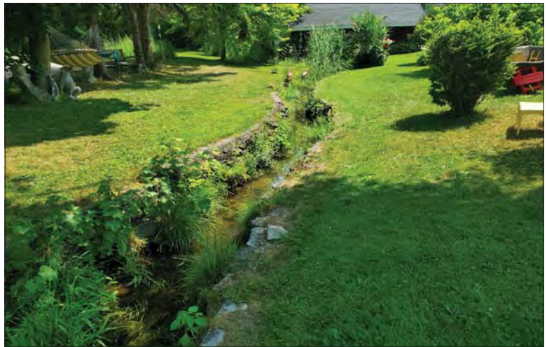
WILLS Saugeen Conservation Filename: 20230705_112451.jpg Photo 62 - October 26, 2023 Durham Creek Flood Plain Mapping Durham Creek: Garafraxa St S Culvert Looking Upstream
