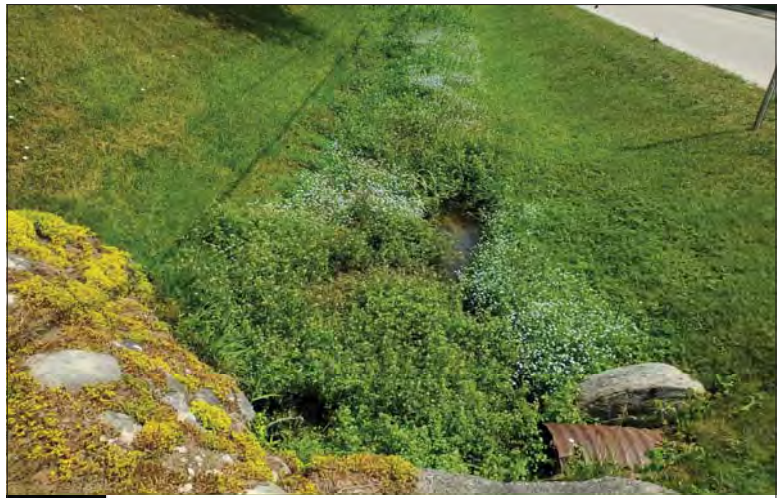
WILLS Saugeen Conservation Filename: 20230705_131944.jpg Photo 86 - October 26, 2023 Durham Creek Flood Plain Mapping Durham Creek: Saddler St E Culvert Looking Upstream
