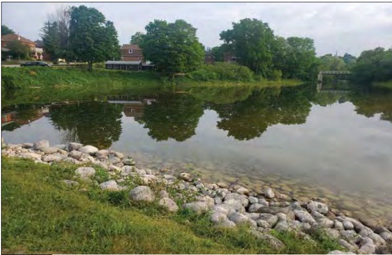
WILLS Saugeen Conservation Filename: 20230706_080236.jpg Photo 143 - October 26, 2023 Durham Creek Flood Plain Mapping Saugeen River: Lower Durham Dam Reservoir
