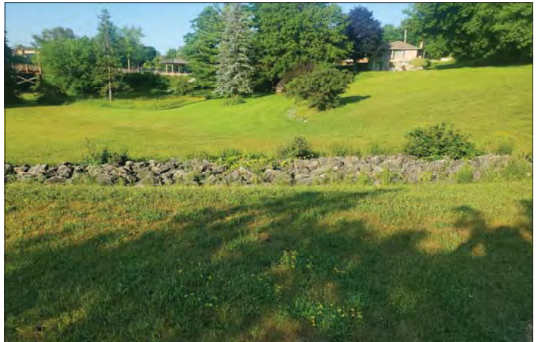
WILLS Saugeen Conservation Filename: 20230707_080215.jpg Photo 238 - October 26, 2023 Durham Creek Flood Plain Mapping Saugeen River: Middle Durham Dam Looking Southwest
