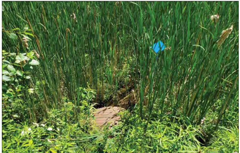
WILLS Saugeen Conservation Filename: 20230707_143944.jpg Photo 118 - October 26, 2023 Durham Creek Flood Plain Mapping Durham Creek: Grey County Rd 4 Culvert Downstream Outlet
