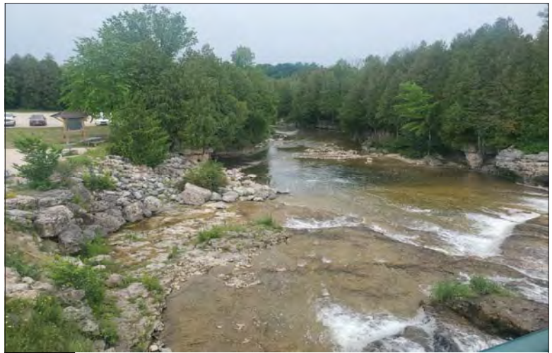
WILLS Saugeen Conservation Filename: 20230706_111638.jpg Photo 290 - October 26, 2023 Durham Creek Flood Plain Mapping Saugeen River: Upper Durham Dam Looking Downstream
