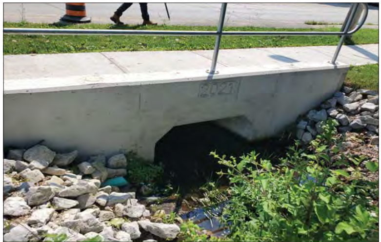
WILLS Saugeen Conservation Filename: 20230705_112548.jpg Photo 64 - October 26, 2023 Durham Creek Flood Plain Mapping Durham Creek: Garafraxa St S Culvert Downstream Face
