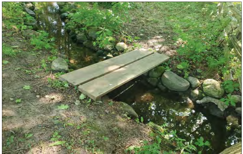
WILLS Saugeen Conservation Filename: 20230705_101114.jpg Photo 52 - October 26, 2023 Durham Creek Flood Plain Mapping Durham Creek: 245 Queen St S Backyard Footbridge Downstream Face
