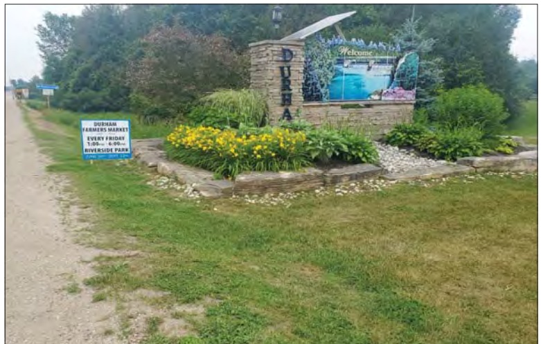
WILLS Saugeen Conservation Filename: 20230706_114202.jpg Photo 348 - October 26, 2023 Durham Creek Flood Plain Mapping Saugeen River: Upper Durham Dam Earth Berm South of Reservoir at End of Berm at Grey County Road 4
