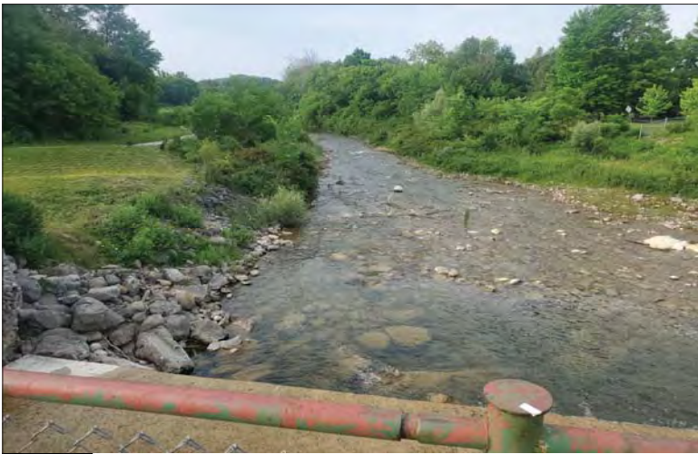
WILLS Saugeen Conservation Filename: 20230706_080202.jpg Photo 139 - October 26, 2023 Durham Creek Flood Plain Mapping Saugeen River: Lower Durham Dam Looking Downstream
