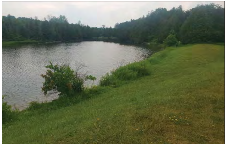
WILLS Saugeen Conservation Filename: 20230706_113318.jpg Photo 334 - October 26, 2023 Durham Creek Flood Plain Mapping Saugeen River: Upper Durham Dam View from Earth Berm
