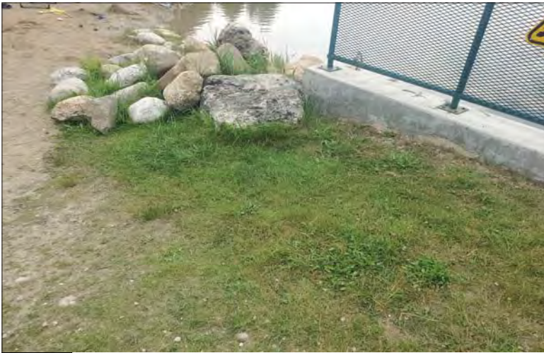
WILLS Saugeen Conservation Filename: 20230706_111945.jpg Photo 311 - October 26, 2023 Durham Creek Flood Plain Mapping Saugeen River: Upper Durham Dam Upstream Wingwall North Bank
