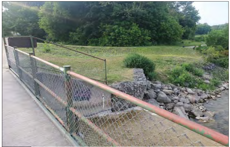
WILLS Saugeen Conservation Filename: 20230706_080206.jpg Photo 140 - October 26, 2023 Durham Creek Flood Plain Mapping Saugeen River: Lower Durham Dam Downstream East Bank
