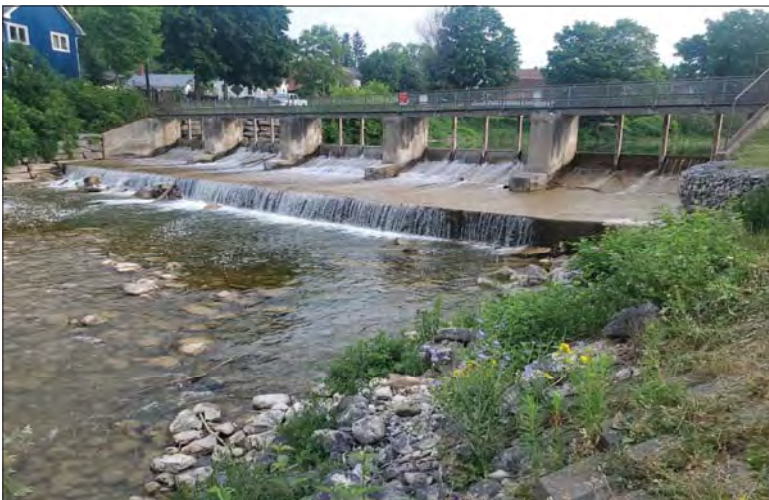
WILLS Saugeen Conservation Filename: 20230706_081002.jpg Photo 167 - October 26, 2023 Durham Creek Flood Plain Mapping Saugeen River: Lower Durham Dam Downstream Face
