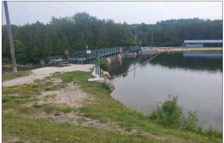
WILLS Saugeen Conservation Filename: 20230706_113127.jpg Photo 322 - October 26, 2023 Durham Creek Flood Plain Mapping Saugeen River: Upper Durham Dam Upstream Side
