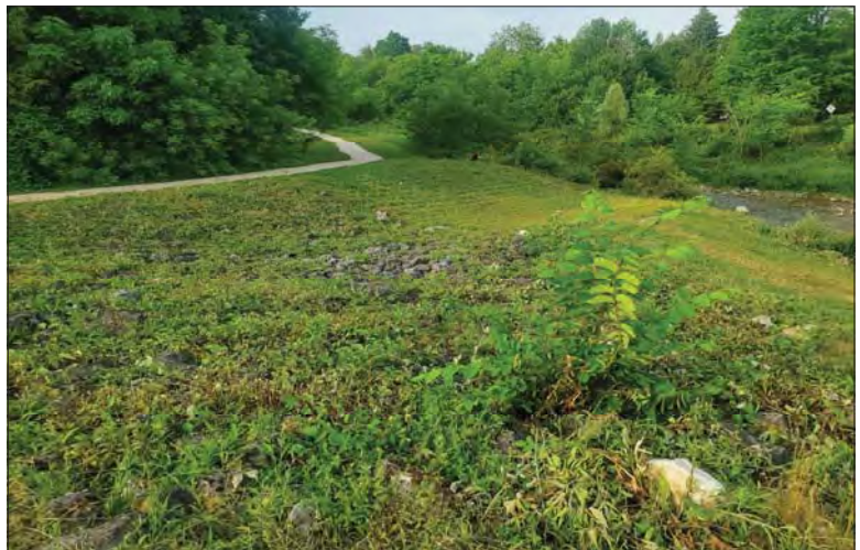
WILLS Saugeen Conservation Filename: 20230706_080249.jpg Photo 148 - October 26, 2023 Durham Creek Flood Plain Mapping Saugeen River: Lower Durham Dam Emergency Spillway
