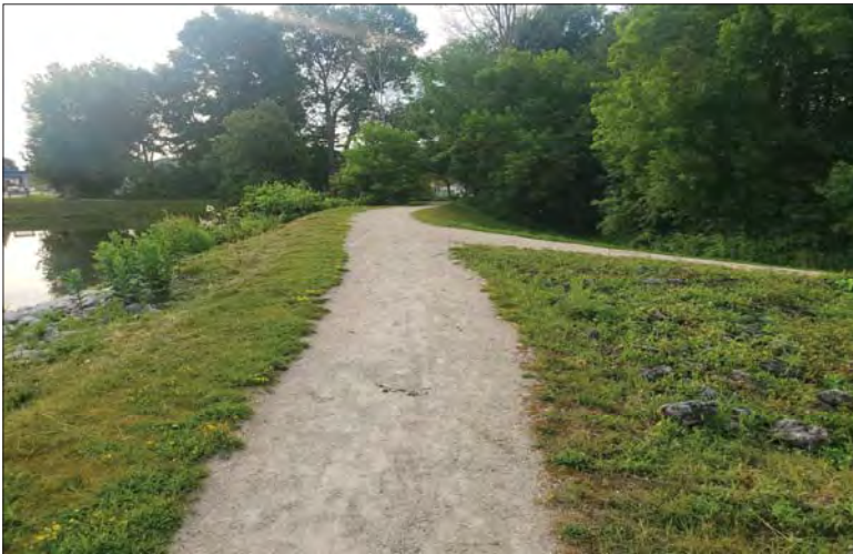
WILLS Saugeen Conservation Filename: 20230706_080227.jpg Photo 141 - October 26, 2023 Durham Creek Flood Plain Mapping Saugeen River: Lower Durham Dam Earth Berm
