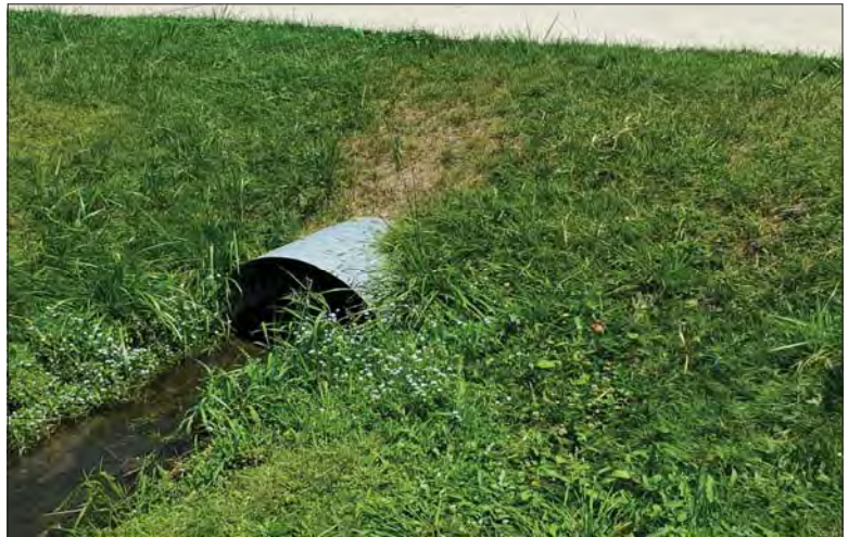
WILLS Saugeen Conservation Filename: 20230704_125833.jpg Photo 10 - October 26, 2023 Durham Creek Flood Plain Mapping Durham Creek: 274 South St W Driveway Downstream Face
