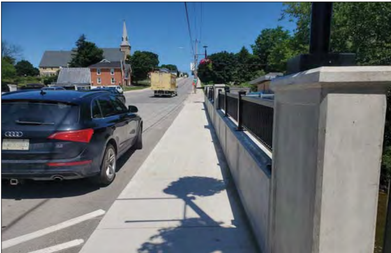
WILLS Saugeen Conservation Filename: 20230707_122842.jpg Photo 201 - October 26, 2023 Durham Creek Flood Plain Mapping Saugeen River: Highway 6 Bridge South Abutment Looking North
