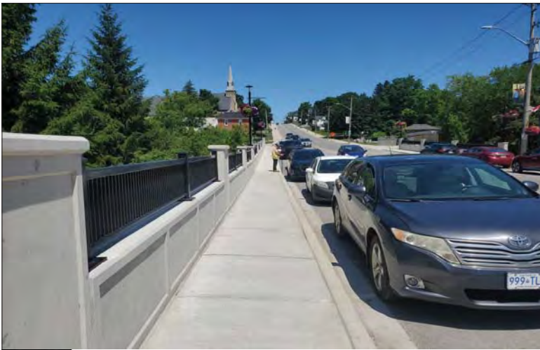
WILLS Saugeen Conservation Filename: 20230707_122940.jpg Photo 199 - October 26, 2023 Durham Creek Flood Plain Mapping Saugeen River: Highway 6 Bridge South Abutment Looking North
