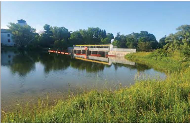
WILLS Saugeen Conservation Filename: 20230707_080256.jpg Photo 235 - October 26, 2023 Durham Creek Flood Plain Mapping Saugeen River: Middle Durham Dam Upstream Face
