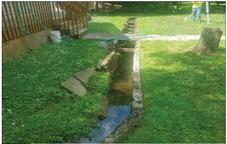
WILLS Saugeen Conservation Filename: 20230704_155813.jpg Photo 32 - October 26, 2023 Durham Creek Flood Plain Mapping Durham Creek: 265 Queen St S Backyard Channel Looking Upstream
