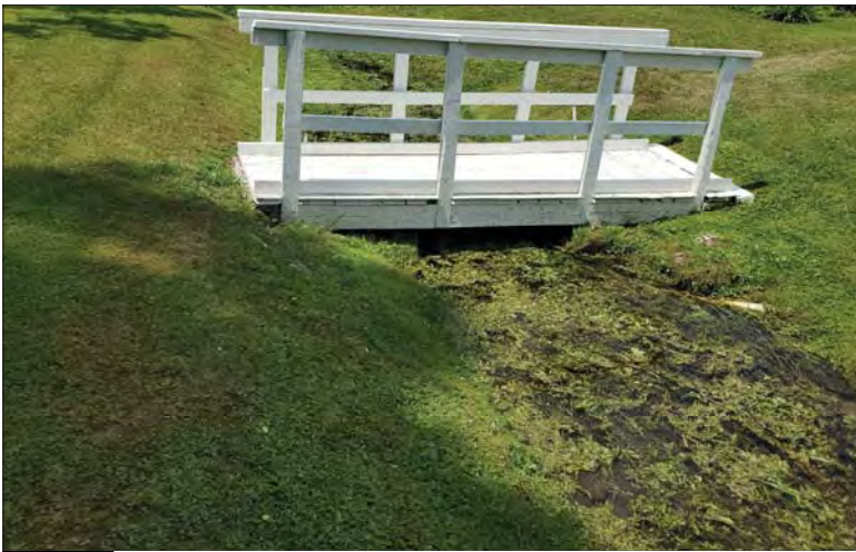
WILLS Saugeen Conservation Filename: 20230705_131036.jpg Photo 73 - October 26, 2023 Durham Creek Flood Plain Mapping Durham Creek: 197 Saddler St E Backyard Footbridge Upstream Face
