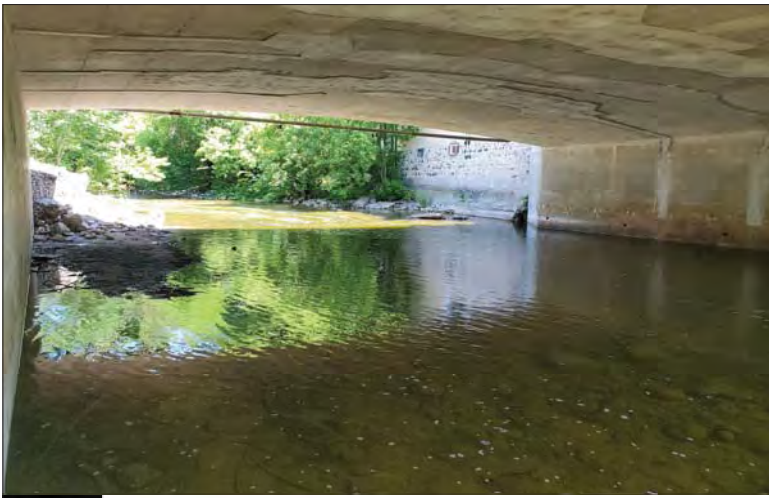
WILLS Saugeen Conservation Filename: 20230707_134007.jpg Photo 205 - October 26, 2023 Durham Creek Flood Plain Mapping Saugeen River: Highway 6 Bridge Soffit Looking Upstream
