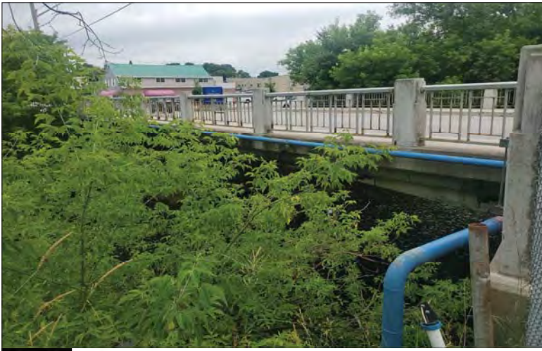
WILLS Saugeen Conservation Filename: 20230706_170811.jpg Photo 177 - October 26, 2023 Durham Creek Flood Plain Mapping Saugeen River: Lambton St E Bridge Upstream Face
