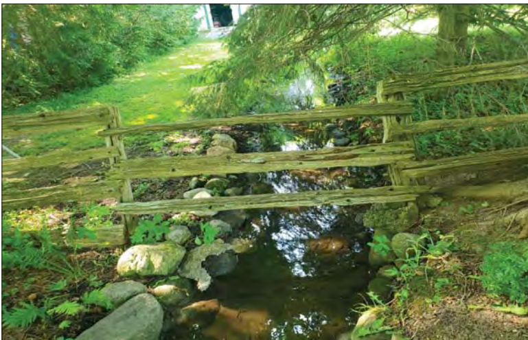
WILLS Saugeen Conservation Filename: 20230705_101104.jpg Photo 51 - October 26, 2023 Durham Creek Flood Plain Mapping Durham Creek: 245 Queen St S Backyard Footbridge Looking Downstream
