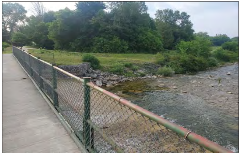
WILLS Saugeen Conservation Filename: 20230706_080121.jpg Photo 134 - October 26, 2023 Durham Creek Flood Plain Mapping Saugeen River: Lower Durham Dam Downstream East Bank
