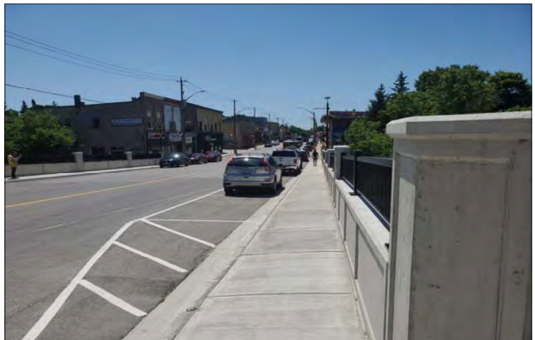
WILLS Saugeen Conservation Filename: 20230707_122612.jpg Photo 196 - October 26, 2023 Durham Creek Flood Plain Mapping Saugeen River: Highway 6 Bridge North Abutment Looking South
