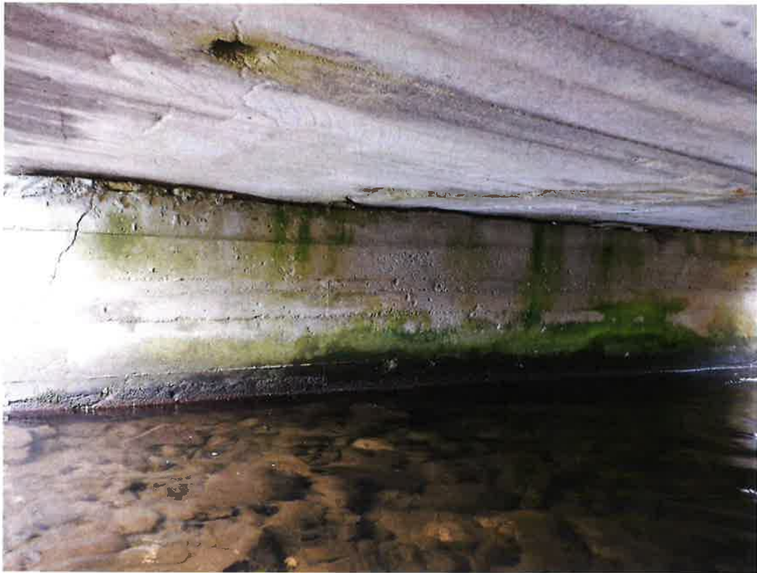
Photograph 3 – South Abutment – Note the gap at the slab/abutment juncture.
