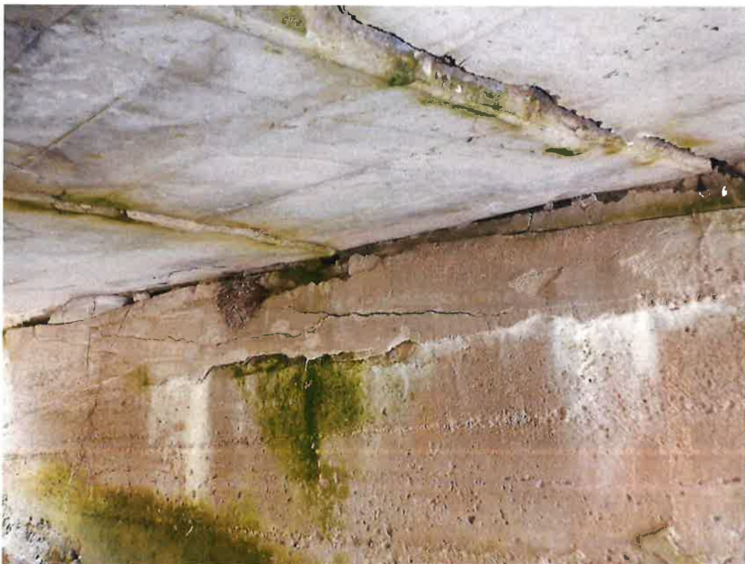
Photograph 4 – Close-up of the north abutment. Note the cracking of the concrete in the abutment and the longitudinal cracks in the deck.
