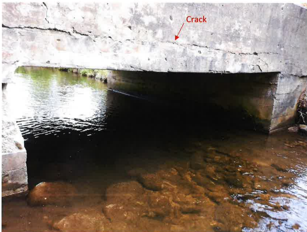
Photograph 8 – West elevation. Note the deterioration and cracking of the structure slab.
