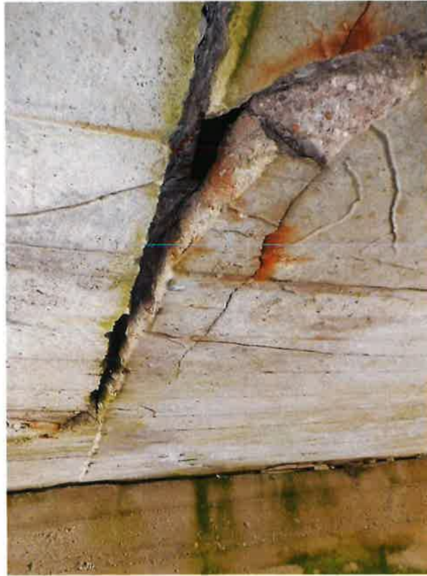
Photograph 5 – Longitudinal cracks in deck slab soffit looking south.
