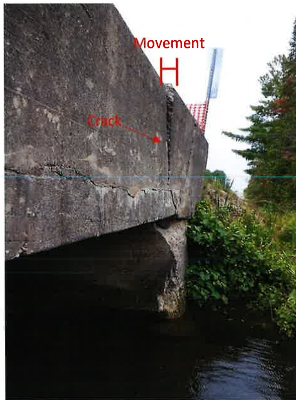
Photograph 9 – Broken wall at northeast corner.
