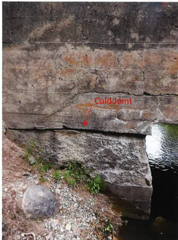
Photograph 7 – Deterioration on the northwest corner. Note the depth of the scaling with no visible reinforcement.
