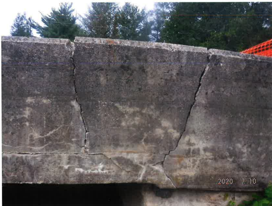
Photograph 10 – East wall at north end of span. Note the v-shaped wedge on the wall that has partially dislodged from the wall.
