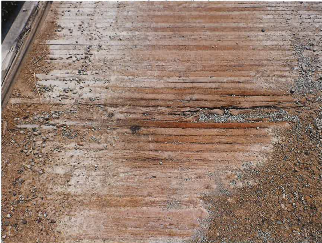
Photograph 6 – Worn and deteriorating wooden deck surface
