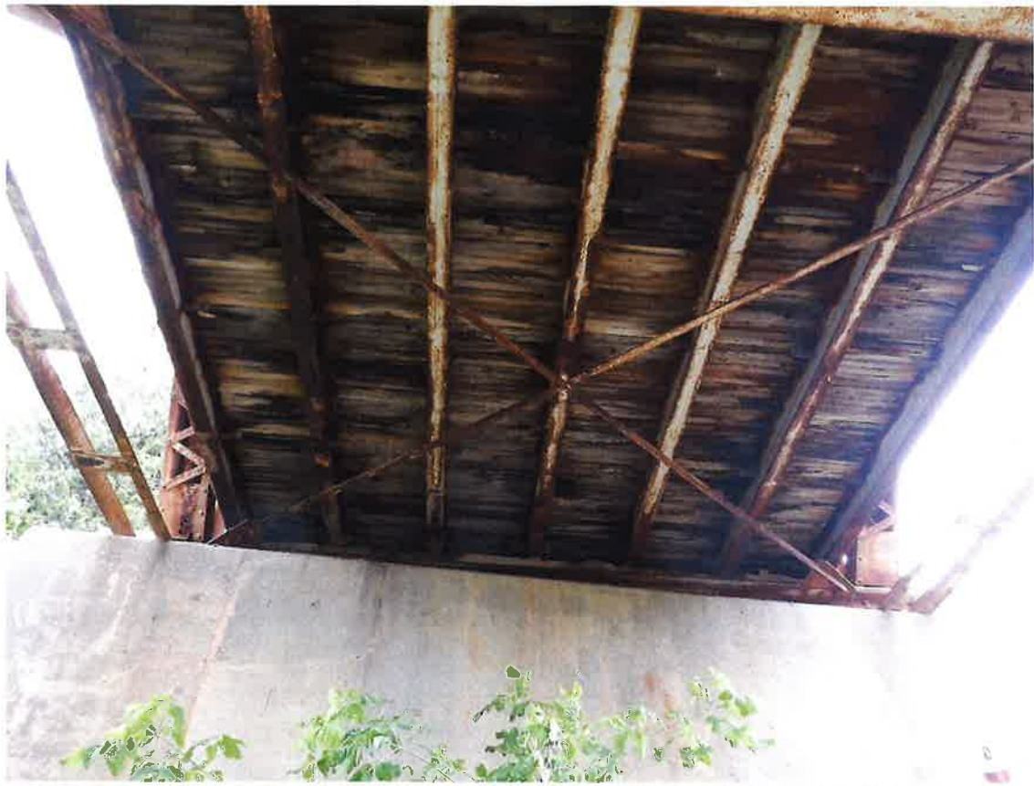
Photograph 11 – Areas of deck soffit with noticeably wet and dark areas indicating decay is present
