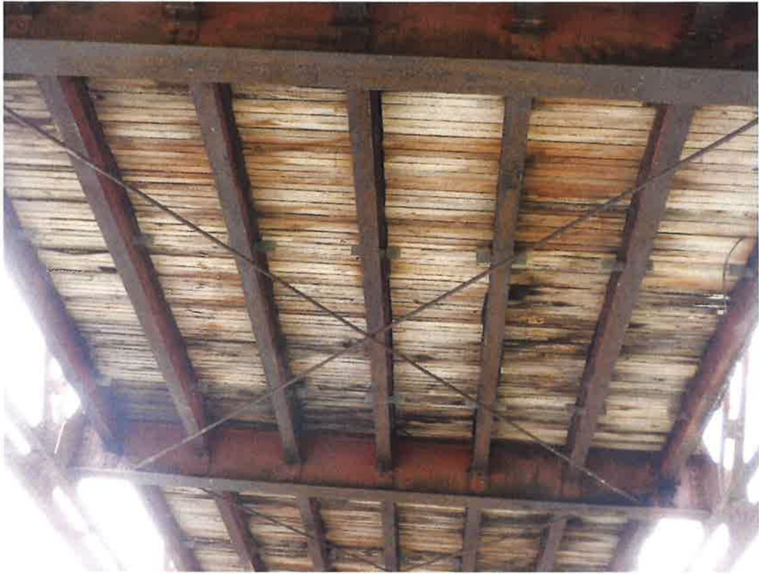
Photograph 5 – Stringers running along deck soffit to floor beams and pier
