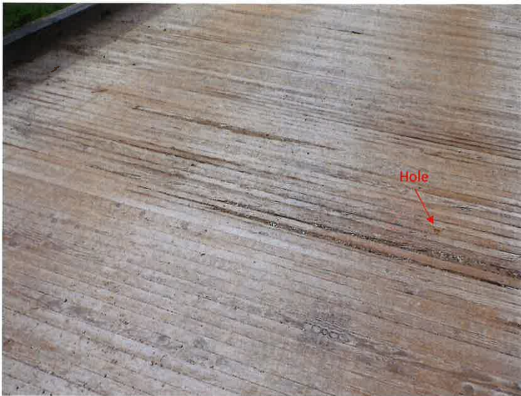
Photograph 9 – Area which deform noticeably under the weight of an inspector
