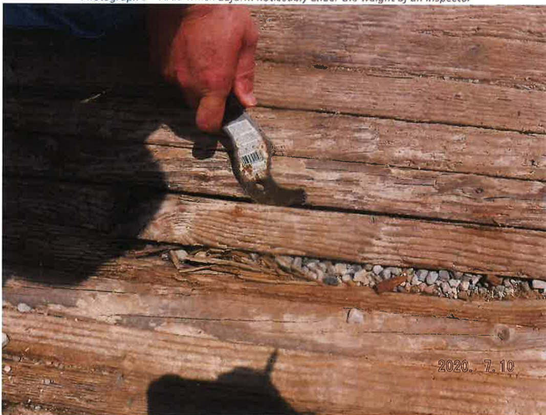
Photograph 10 – Laminate deck can be easily separated with a paint scraper
