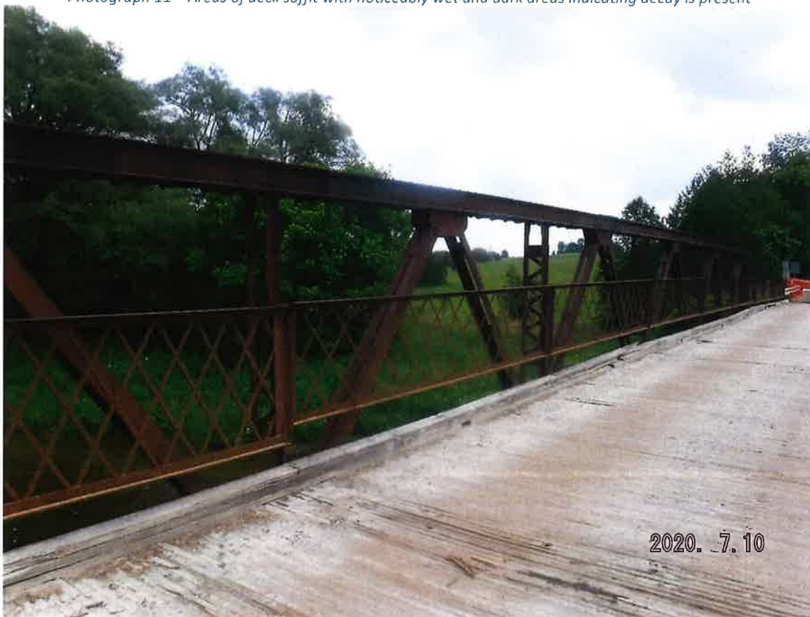
Photograph 12 – East pony truss
