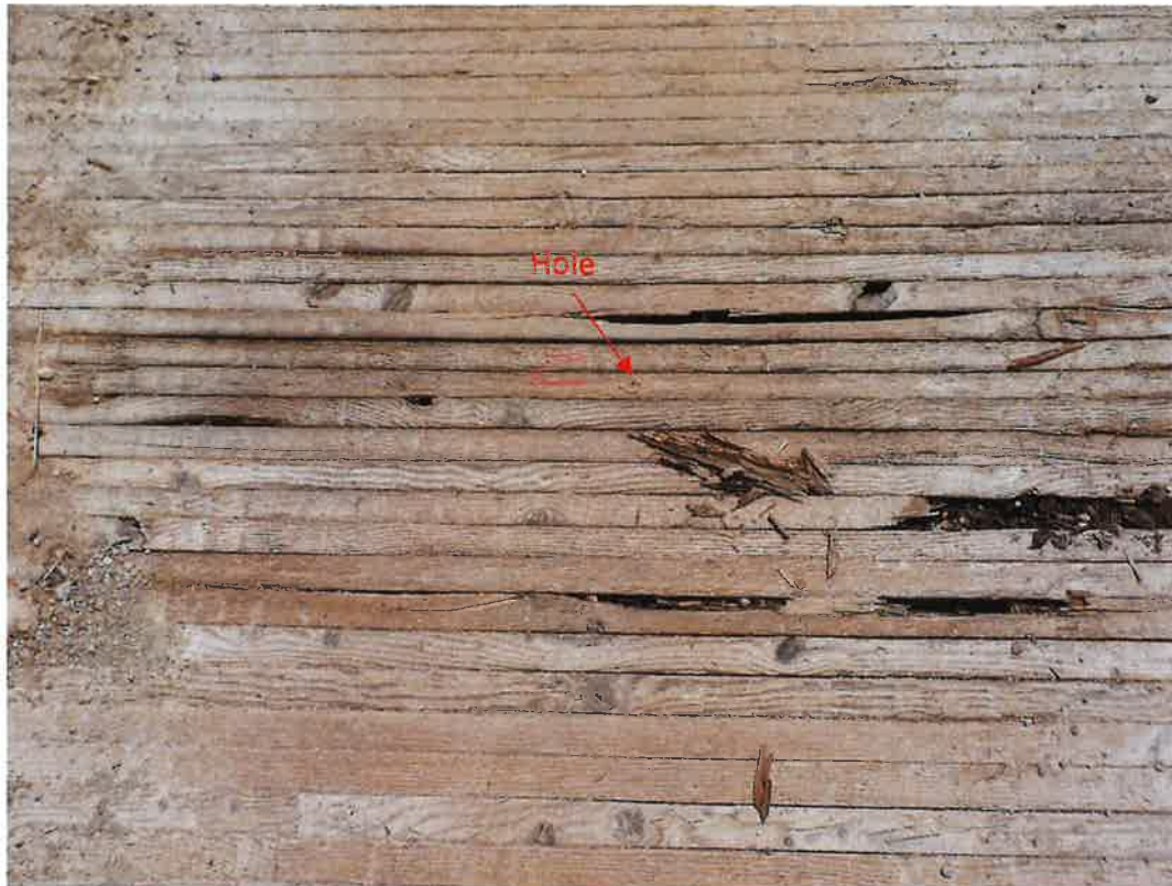
Photograph 7 – Deck surface with broken/deteriorating laminate
