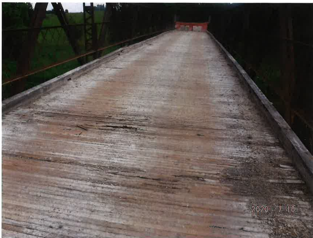
Photograph 3 – Deck made of 2"x6" sawn timbers (transverse laminated)
