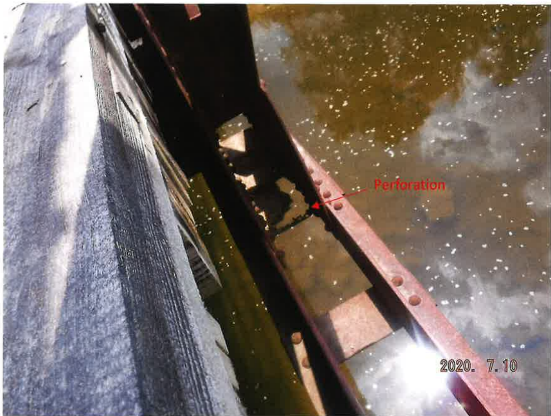
Photograph 13 – Corroded/perforated connection plate on bottom chord
