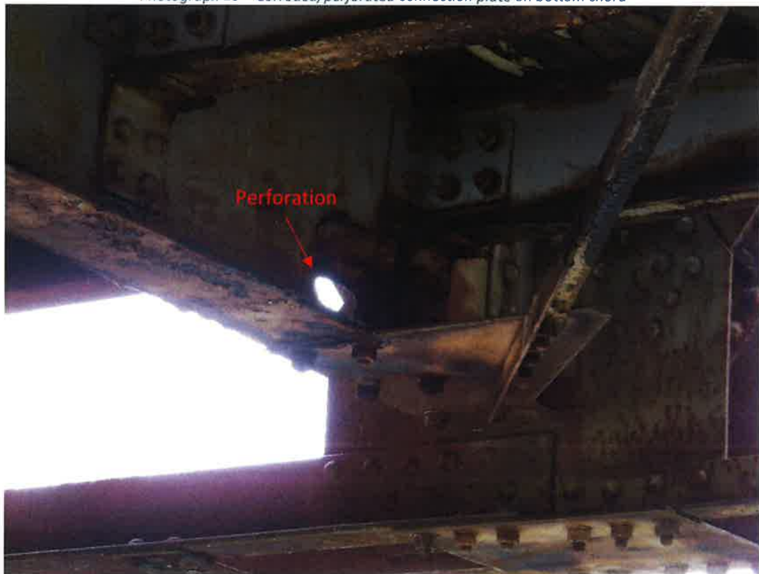
Photograph 14 – Perforation in floor beam web in NW corner
