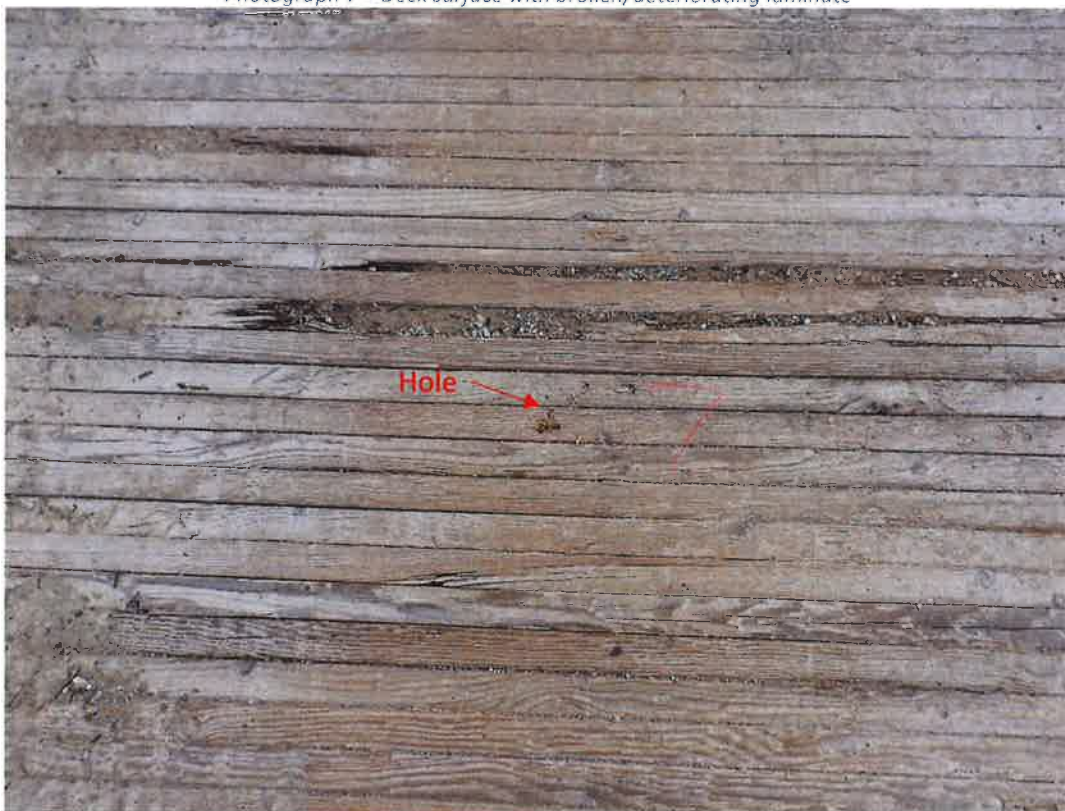
Photograph 8 – Drilling into wooden deck to confirm state of decay indicated by hammer sounding
