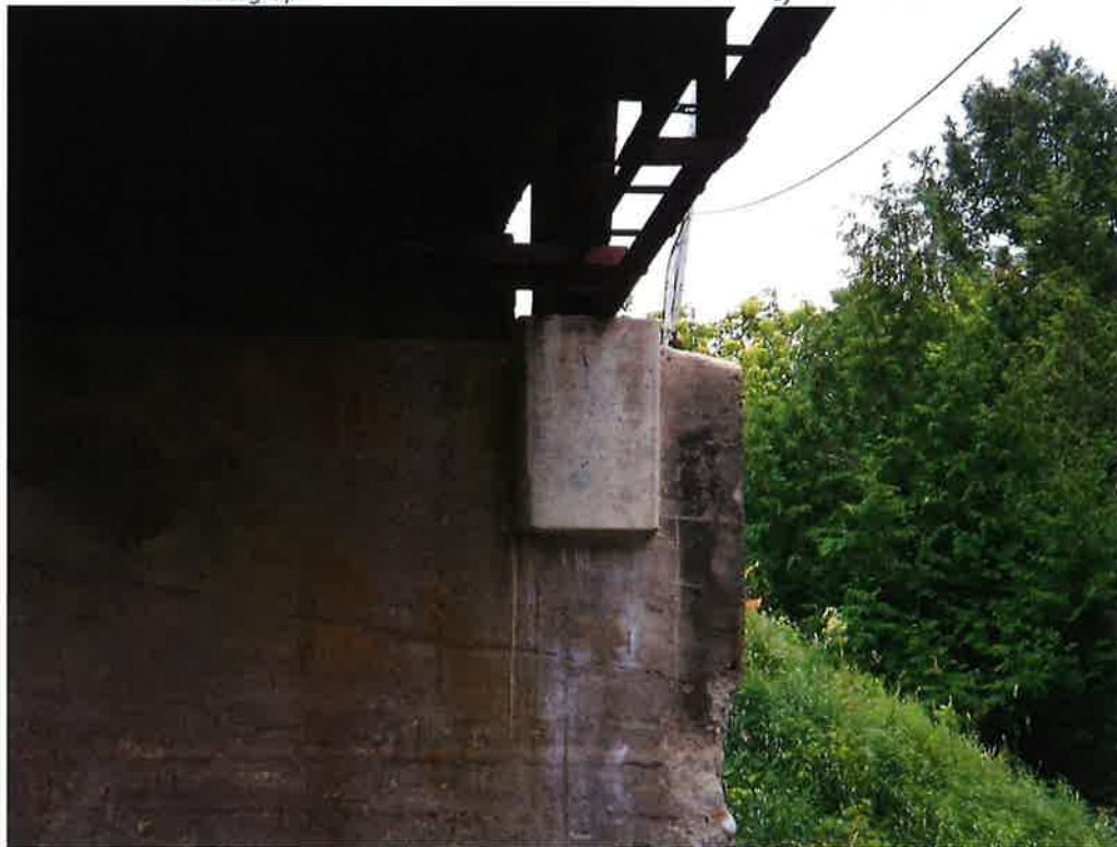
Photograph 16 – Corbel indicating some modifications to the pier (north face west of end pier)
